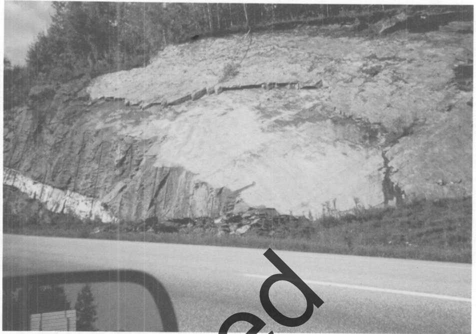
Figure 5.20 A planar joint surface. The surface is macro smooth.
