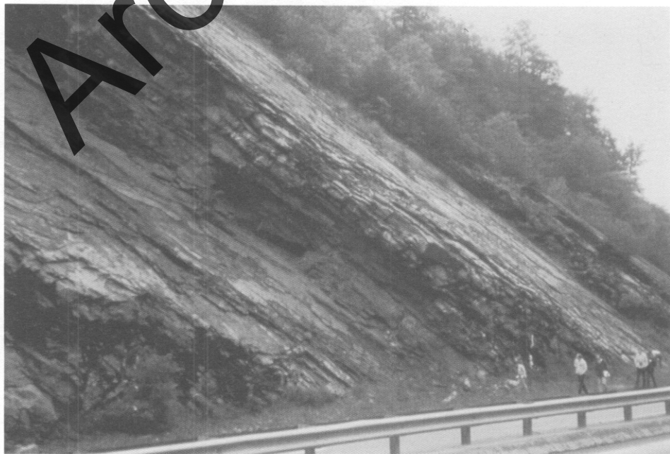
Figure 5.17 Continuous joints with adverse orientation.
