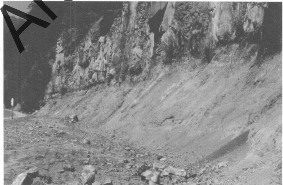
Figure 3.2 "B" rated slope.
