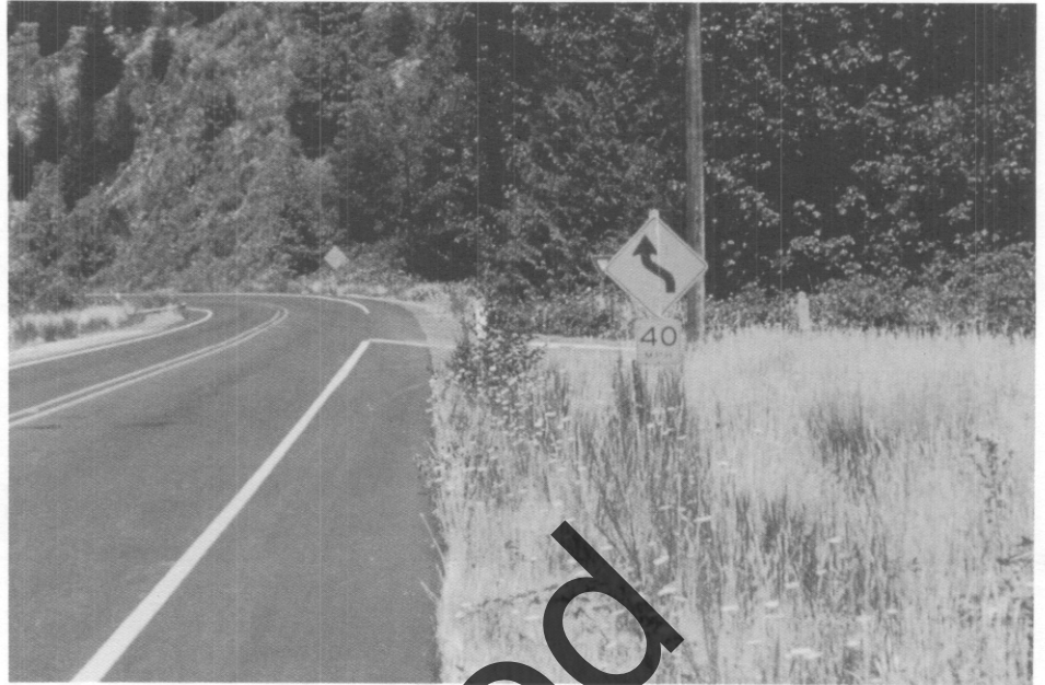
Figure 5.8 Roadway curves with reduced posted speed limits are common in rugged terrain. Remember to record this information.
