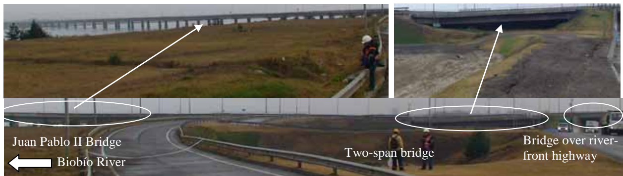
Figure 59. Photo. Approaches to Juan Pablo II bridge.
