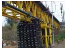
Figure 173. Photo. South end of Chepe railroad bridge.
