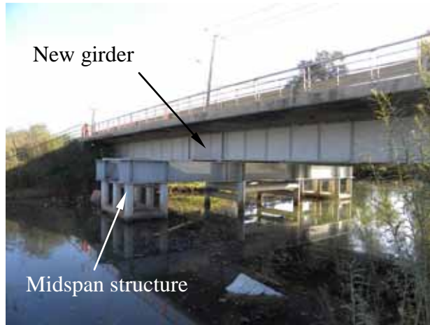
Figure 149. Photo. Side view of El Bar bridge.
