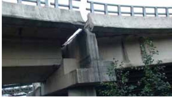
Figure 49. Photo. Exterior face of westbound ramp to Llacolen bridge at the river end.
