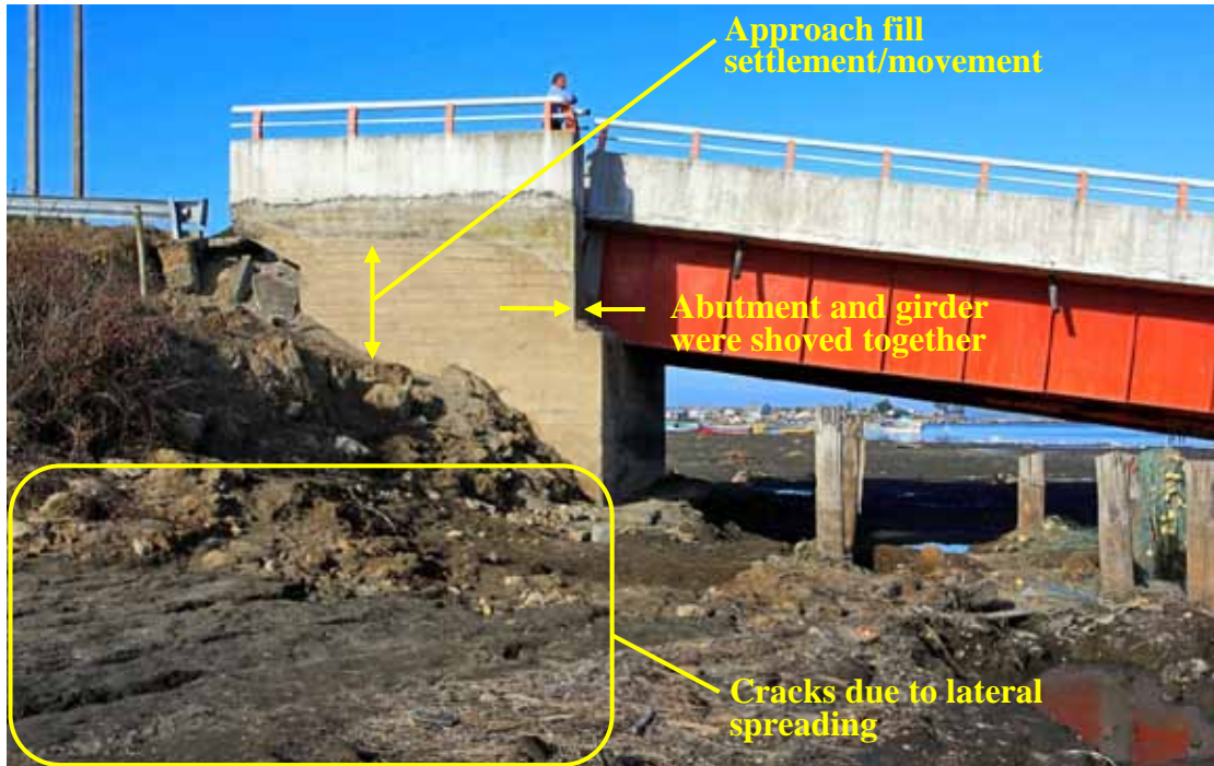
Figure 240. Photo. Overview of Tubul bridge north abutment.
