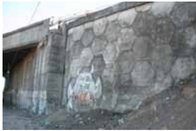
Figure 258. Photo. Retaining wall at 21 de Mayo.
