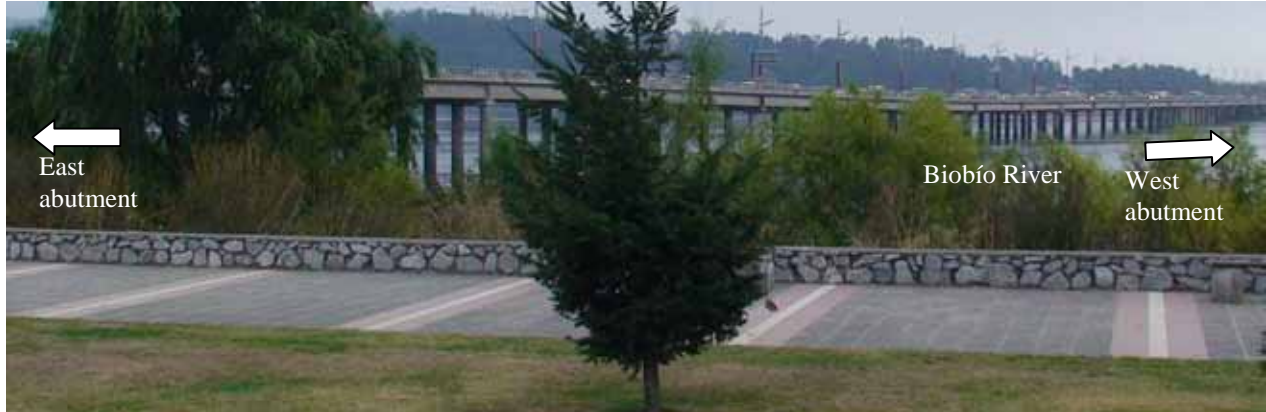
Figure 42. Photo. Llacolen bridge looking south-southwest.
