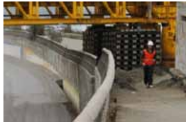
Figure 254. Photo. Retaining wall at Chepe railroad bridge over Biobío River.
