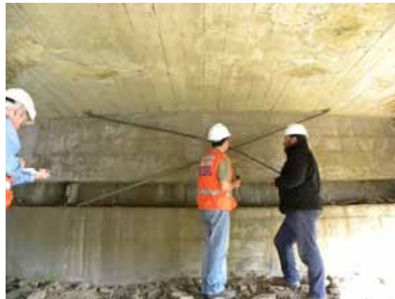
Figure 154. Photo. Damage to rebar X-brace system on north abutment of El Bar bridge.
