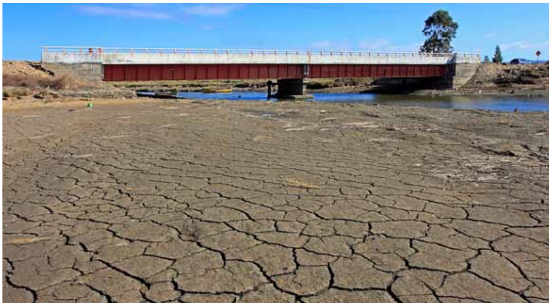
Figure 207. Photo. Raqui 1 bridge viewed from north side.
