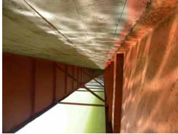
Figure 142. Photo. Web stiffeners in Pichibudis bridge.
