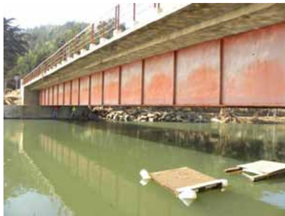
Figure 141. Photo. Cross frames in Pichibudis bridge.
