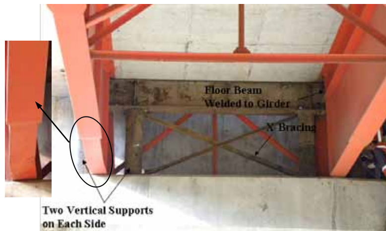
Figure 128. Photo. Temporary repair at northeast abutment of Cardenal Raúl Silva Henríquez bridge
