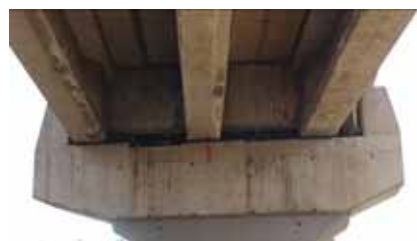
Figure 34. Photo. Flared wall pier of exit ramp from westbound Independencia bridge.
