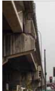
Figure 31. Photo. Westbound Independencia bridge.
