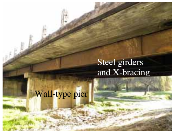
Figure 77. Photo. Overview of west Ramadillas bridge.
