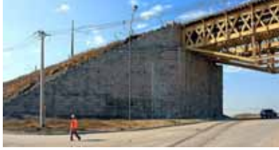
Figure 252. Photo. Retaining wall at Maipú River bridge.
