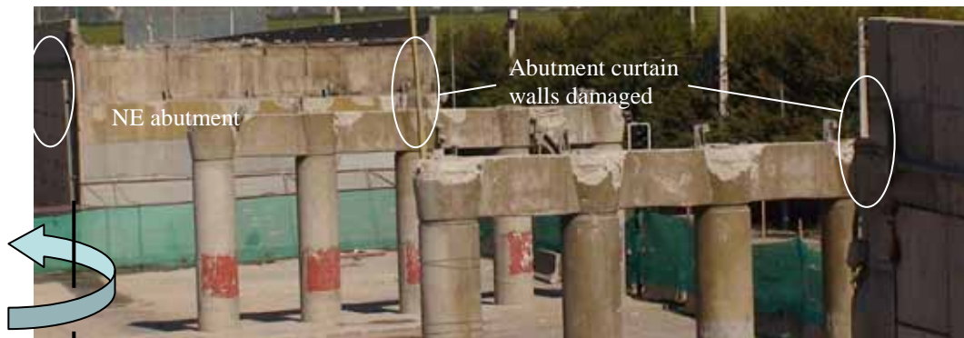
Figure 89. Photo. Miraflores bridge after removal of superstructure.
