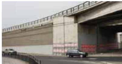
Figure 250. Photo. Retaining wall at Américo Vespucio/Independencia eastbound.
