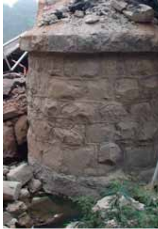
Figure 169. Photo. Foundation of Claro River bridge.
