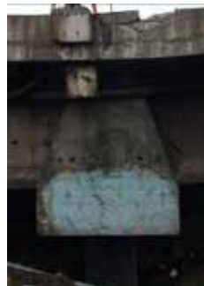
Figure 62. Photo. Intermediate bent of northern approach to Juan Pablo II bridge.
