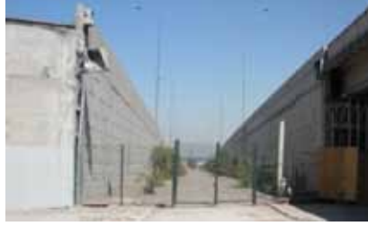
Figure 247. Photo. Retaining wall at Américo Vespucio/Lo Echevers.
