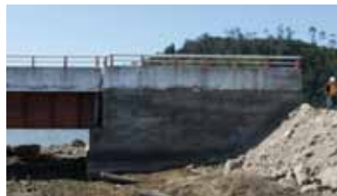
Figure 255. Photo. Retaining wall at Raqui 2.
