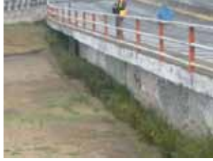
Figure 257. Photo. North retaining wall at Juan Pablo II.
