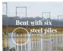
Figure 172. Photo. River spans of Chepe railroad bridge.
