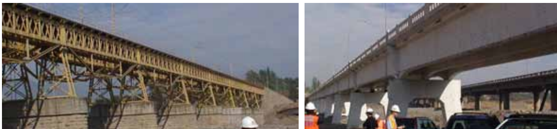
Figure 181. Photo. Three parallel bridges crossing Maipú River south of Santiago.
