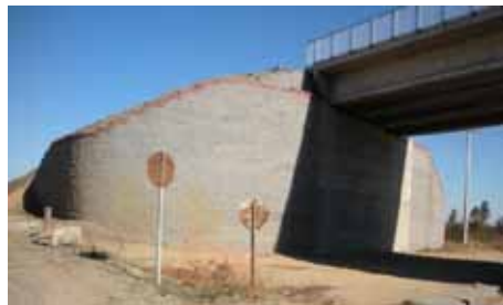
Figure 260. Photo. Retaining wall at Muros Talca (SW).
