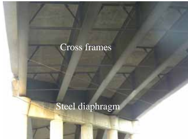
Figure 107. Photo. Cross frames on Quilicura railway overcrossing.
