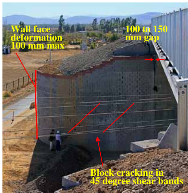
Figure 275. Photo. Wall with steep top slope at Muros Talca.
