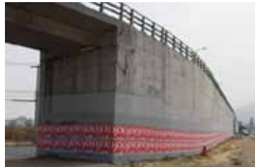
Figure 251. Photo. Retaining wall at Américo Vespucio/Independencia westbound.
