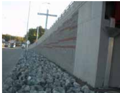
Figure 259. Photo. Retaining wall at Rotonda General Bonilla.
