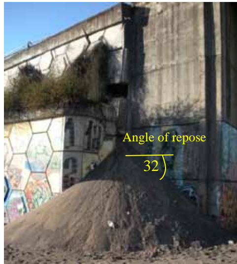
Figure 271. Photo. Fill material from tiered wall at wall site 28C.
