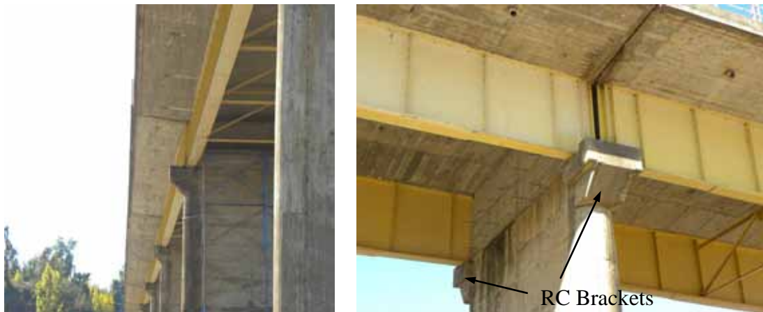
Figure 158. Photo. Girder supports at each pier of Itata River bridge.
