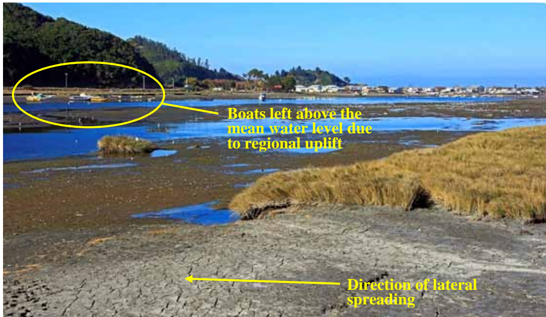
Figure 244. Photo. View northeast from Tubul bridge south abutment showing areas left dry and boats left above the new mean water level.
