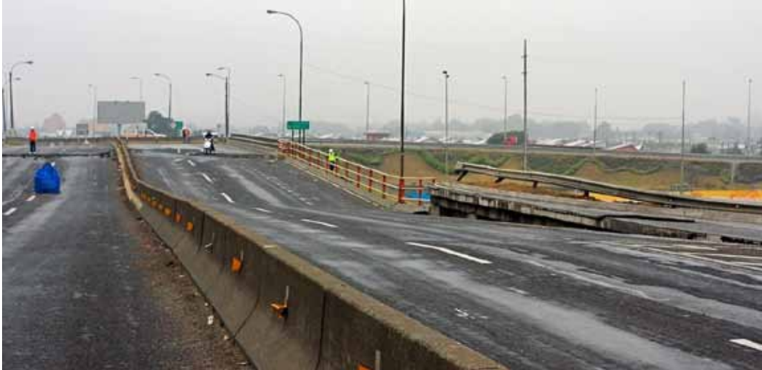
Figure 219. Photo. Roadway settlement due to settlement of approach structure pier foundations for Juan Pablo II bridge.
