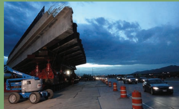
Prefabricated I-15 bridge at Pioneer Crossing in UT.
