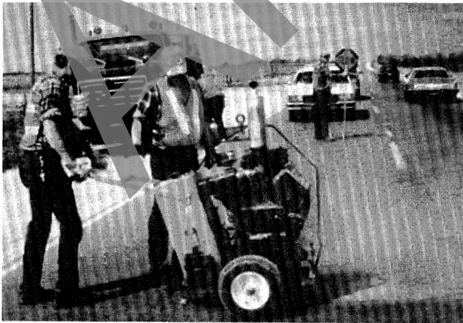
This slide shows a diamond-blade crack saw.
