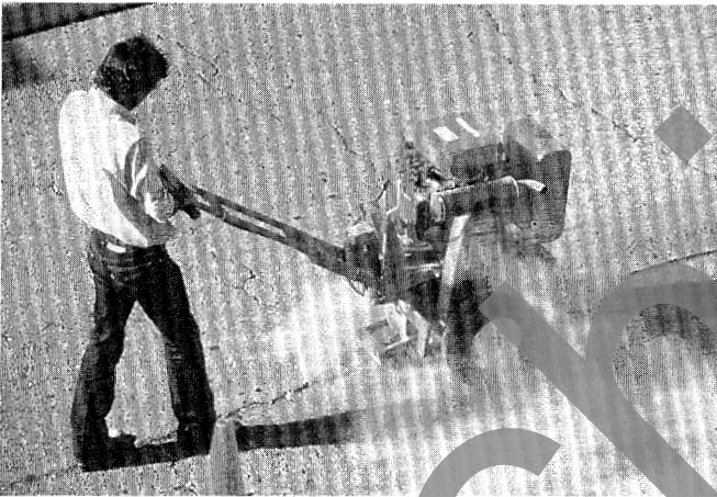
This slide shows a rotary-impact router.
