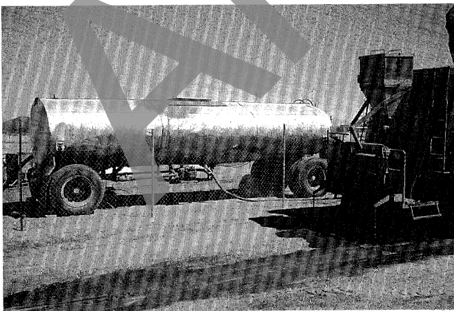
Emulsion being added to the slurry machine.
