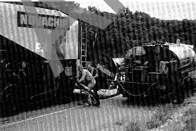
This photo shows nurse trucks used to periodically fill the emulsion tank on the machine. Emulsion tank capacity on these machines is about 8,300 liters; adequate for nearly 3 hours of operation. Emulsion is applied at a temperature of 60°C. The emulsion storage tank was not equipped for reheating the emulsion.
