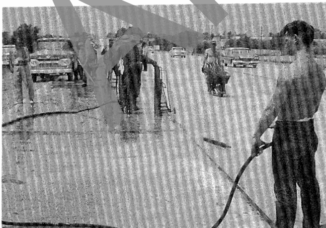
This slide illustrates the process of subsealing.
