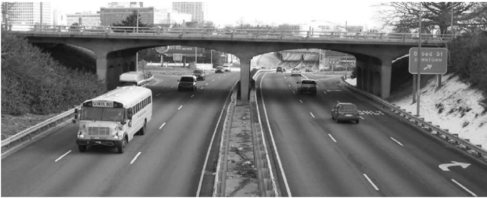
Photo 1. The Broad Street Bridge over US 421 is just one of the many structures needing rehabilitation. The construction skill set recommended replacing the Broad Street Bridge in order to improve vehicle and pedestrian capacity.
