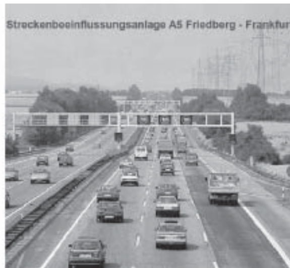
Figure 9. Germany uses variable speed limit and lane status signs in areas with construction or congestion.
