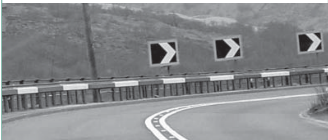
Figure 13. The United Kingdom uses high-performance marking and signing and consistently applied speed limits to improve safety along corridors.
