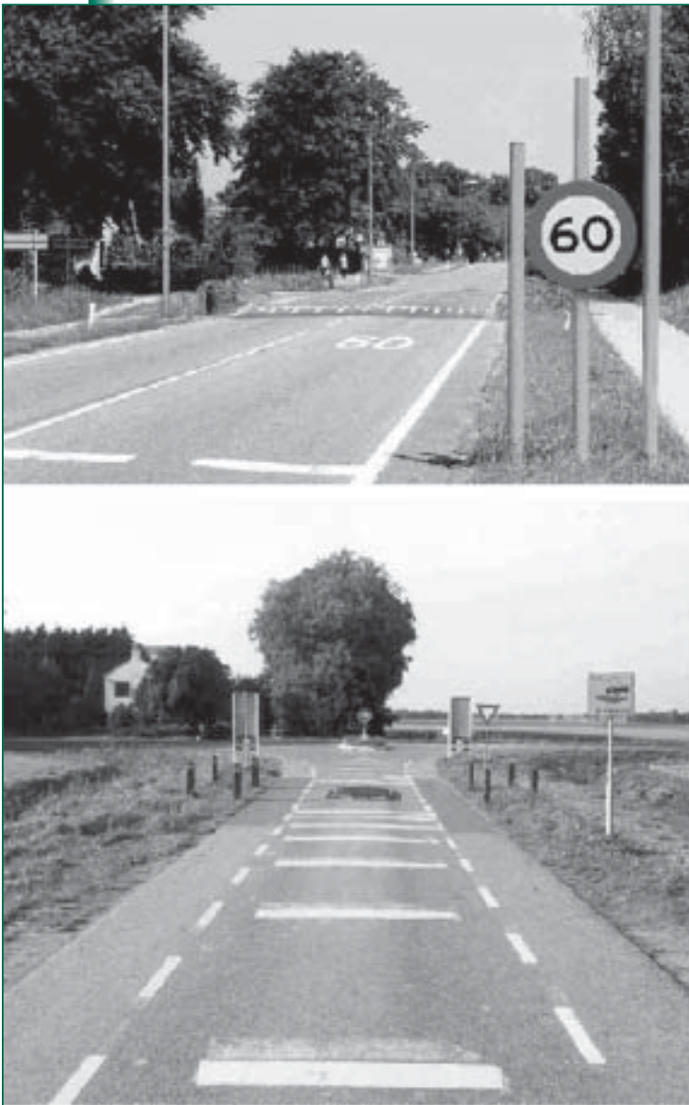
Figure 12. The Netherlands uses self-enforcing roadways and traffic-calming elements to encourage drivers to travel at appropriate speeds.
