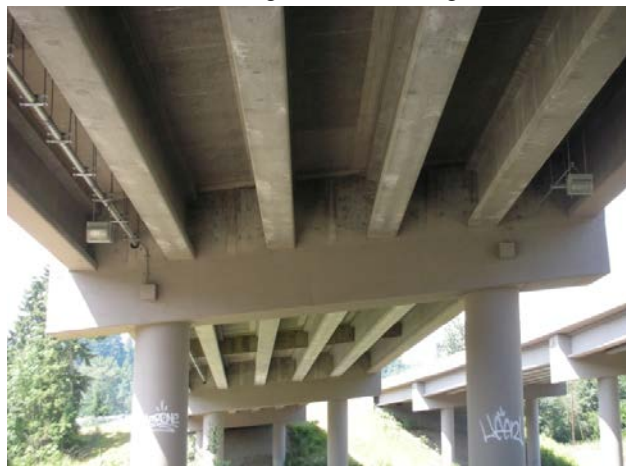
(c) P/S Girders integral with cap
