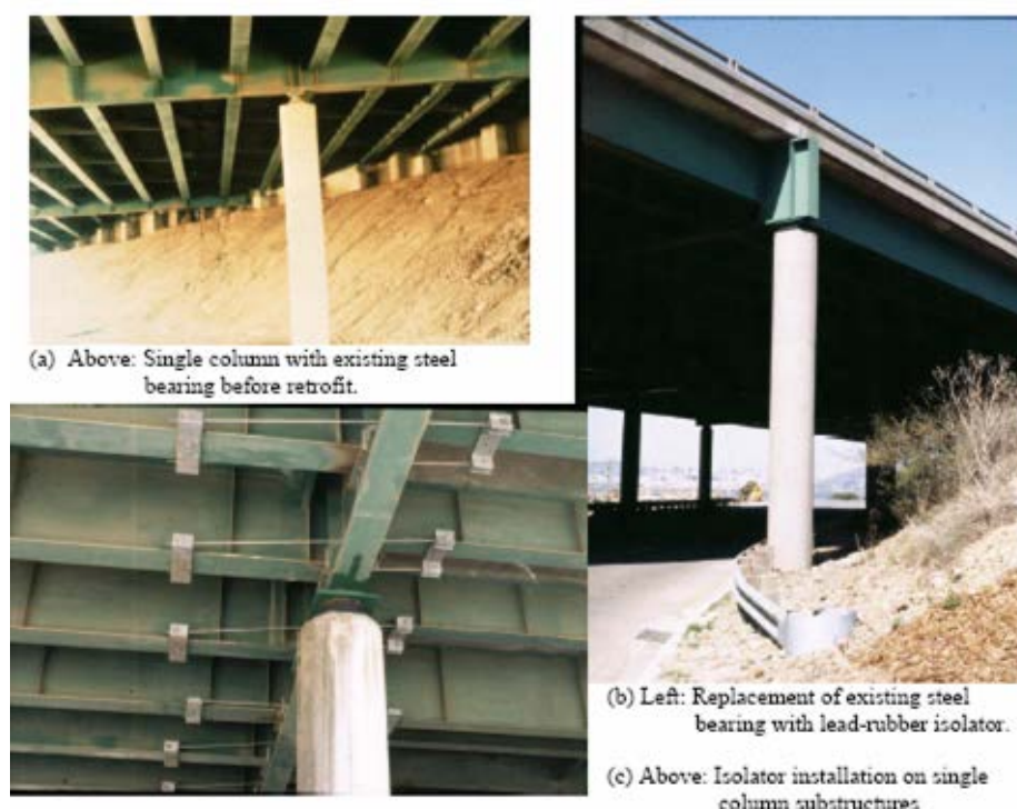
Figure 9-7 Sierra Point Overhead US 101 Near San Francisco (Buckle et. al., 2006)
