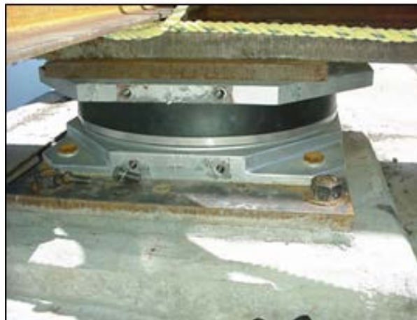
Figure 9-24 Concave Friction Isolator, Mississippi River Bridge, Ontario, Canada (Buckle et.al., 2006)
