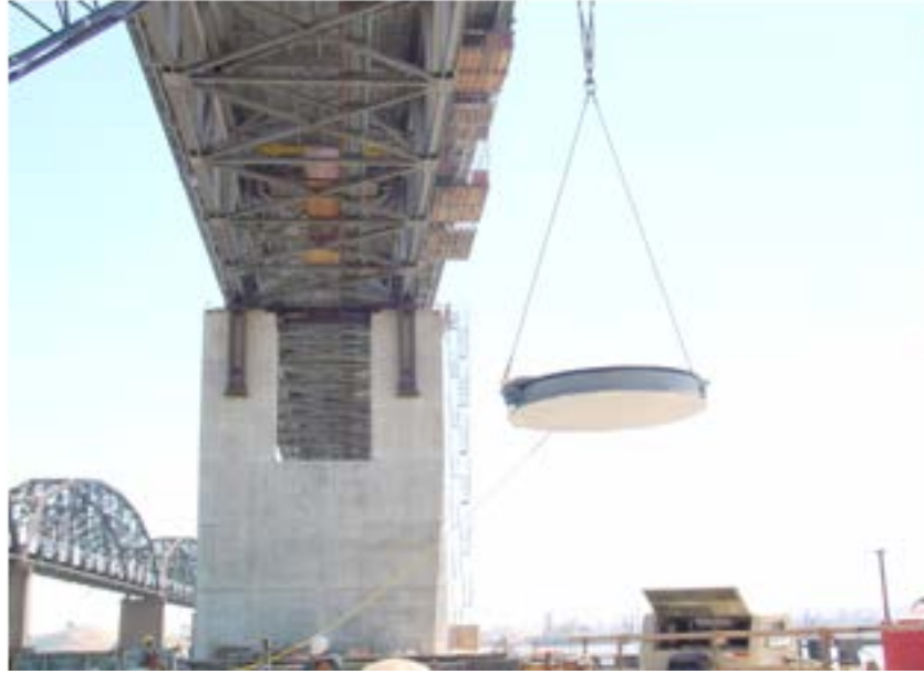
Figure 9-9 Concave Friction Bearings Being Installed in the Benicia-Martinez Bridge, CA
