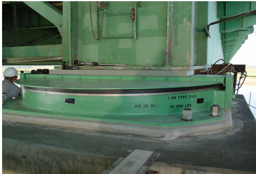
Figure 10-10(d) Lead-Rubber Isolator (top), Friction-Pendulum Isolator (center), and Installation of Friction Pendulum Isolator on I-40 Crossing Mississippi River, Memphis (bottom)
