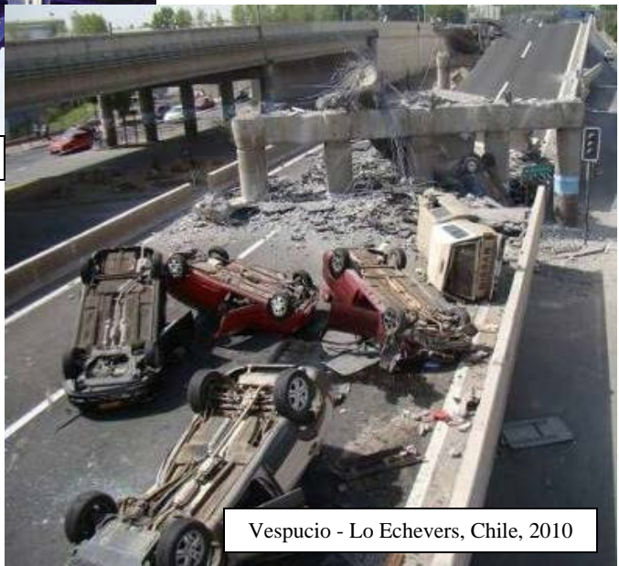
Figure 1-3 Examples of Unseated Spans due to Insufficient Support Length
