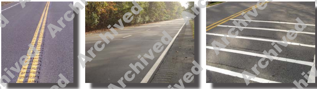
Illustrations of rumble strip for centerline (left), shoulder (middle), and across roadway (right).
