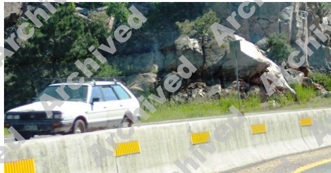
Reflective sheeting shaped to provide linear reflectorization.
