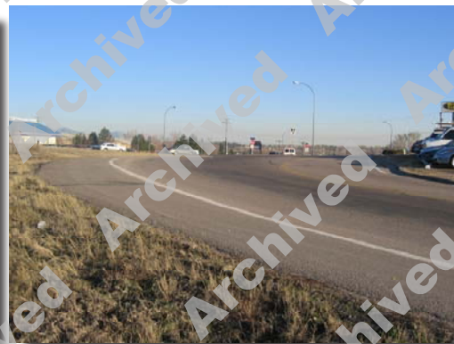
Widening on the outside of the curve.
