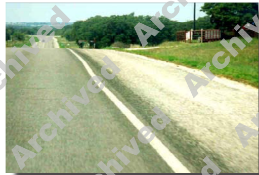
In addition to paving the shoulder, color variation between the shoulder and travel lanes adds visual delineation.
