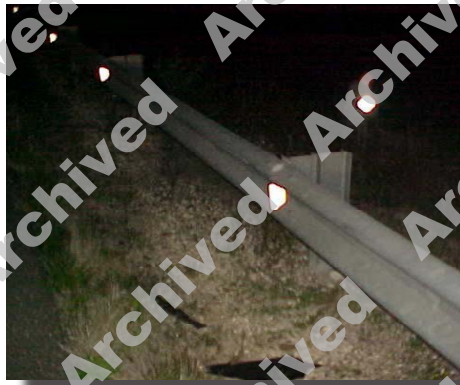
Installation of reflectors on W-beam guardrail.
