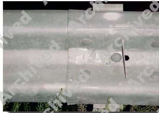
Installation of reflectors on W-beam guardrail.
