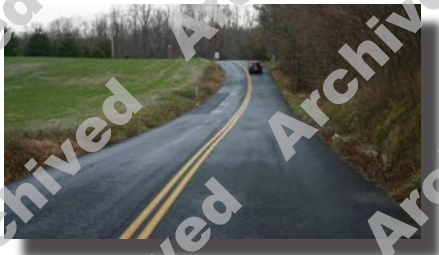
Centerline for No Passing on horizontal curve.
