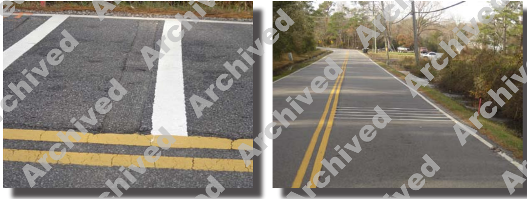
For this RRS application a set of 5 grooves and painted lines were placed 200 ft before the curve.
