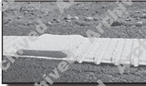
(Source: Caltrans) Raised profile thermoplastic marker.
