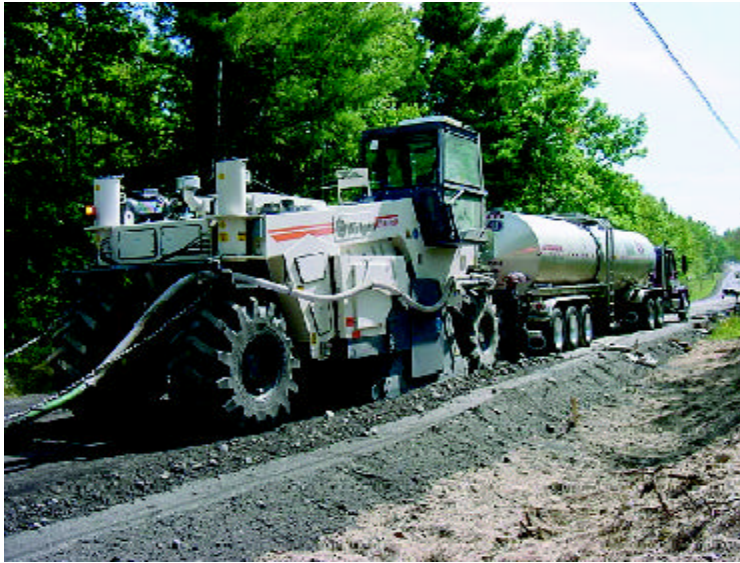
A scan on recycled materials in highway construction in Europe led to a U.S. pilot project on the use of foam bitumen in recycled asphalt.
