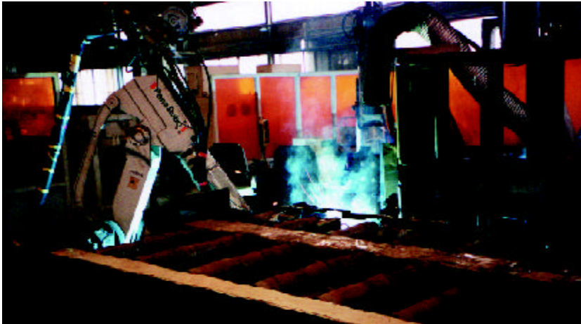
U.S. experts observed the use of automated steel fabrication plants to build high-quality, cost-efficient bridges in Japan.
