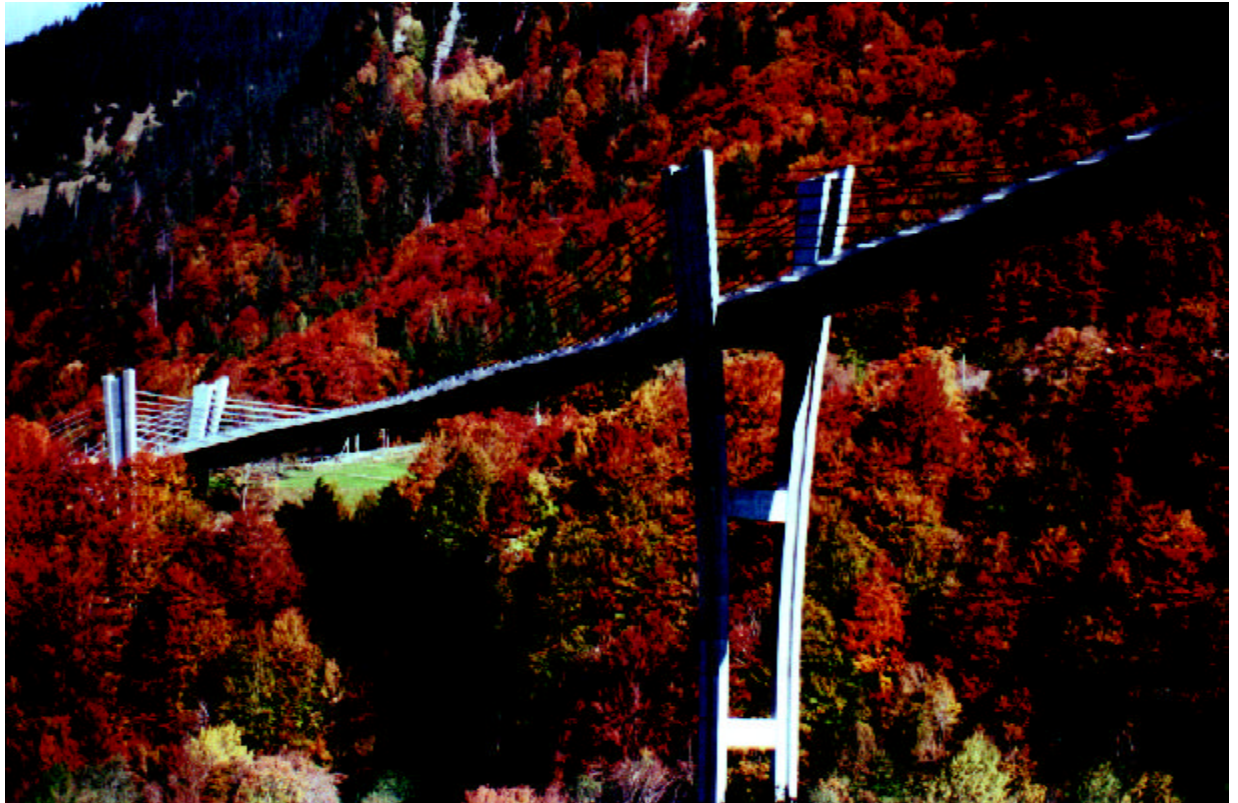
Observing the latest cable-stay bridge technology overseas helps U.S. transportation professionals build aesthetically pleasing, safer and more durable bridges at home.
