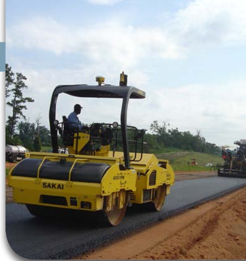
Double drum vibratory steel wheel roller equipped with IC technology
