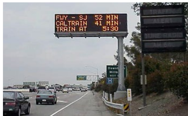
Figure 5. Photo. Comparative freeway and transit travel times on a dynamic message sign in California.
