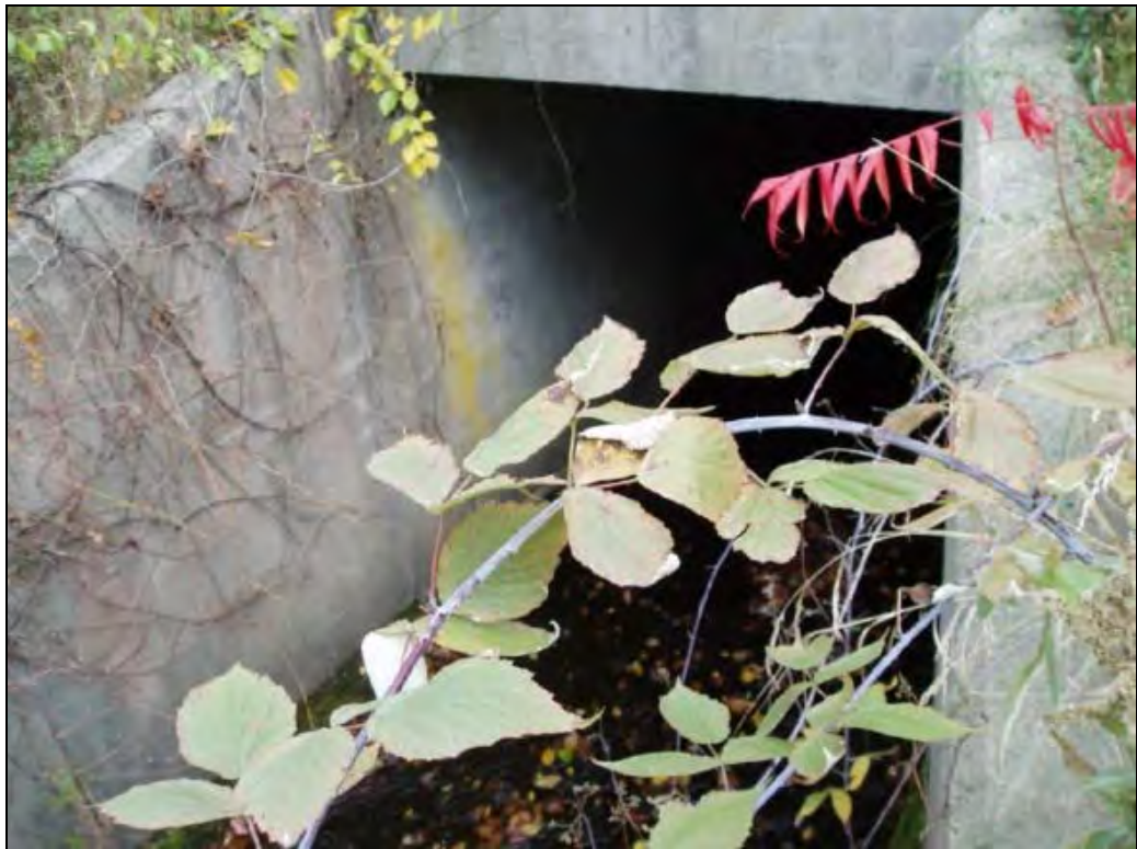
Figure 8.2. Inlet of Bridge 02315.
