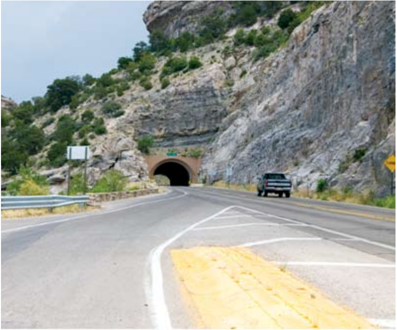
The Cloudcroft Tunnel.
