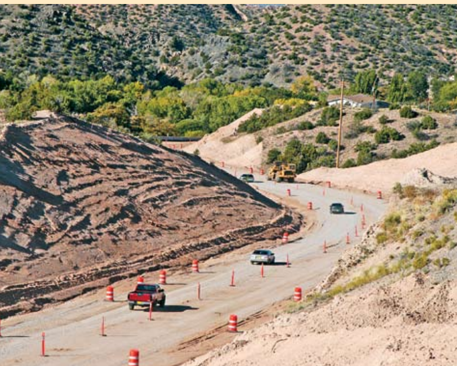
Work on Chimayo Cut.
