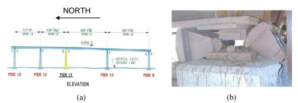
**Figure 2-5** Dunn Memorial Bridge Interchange Rocker Bearing Failure: (a) Sketch of the bridge elevation from Pier 9 to Pier 13; (b) Photo of the failed rocker bearings at Pier 11 showing them tipped over (taken from [29]).
