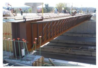
**Figure 2-11** Photo showing the cantilever forming brackets which will support formwork that will be used to construct the concrete deck overhang on a simple span steel girder superstructure.
