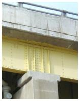
a) Before Rehabilitation b) After Rehabilitation **Figure 2-3** Photos showing the before and after of the elimination of trough-type drainage details by making simple steel spans continuous during a rehabilitation project.
