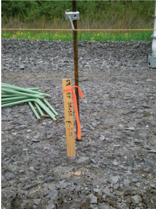
Figure 22 – Surveyed Reference Hub and Stringline
