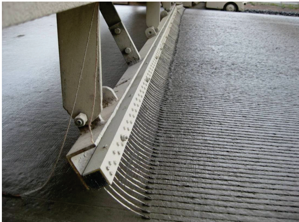
Figure 41 – Clean and Straight Tines Minimizes Positive Texture
