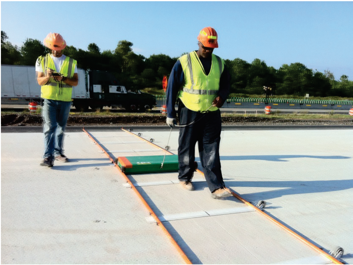
Figure 27 – MIT Scan used to Locate Dowels
