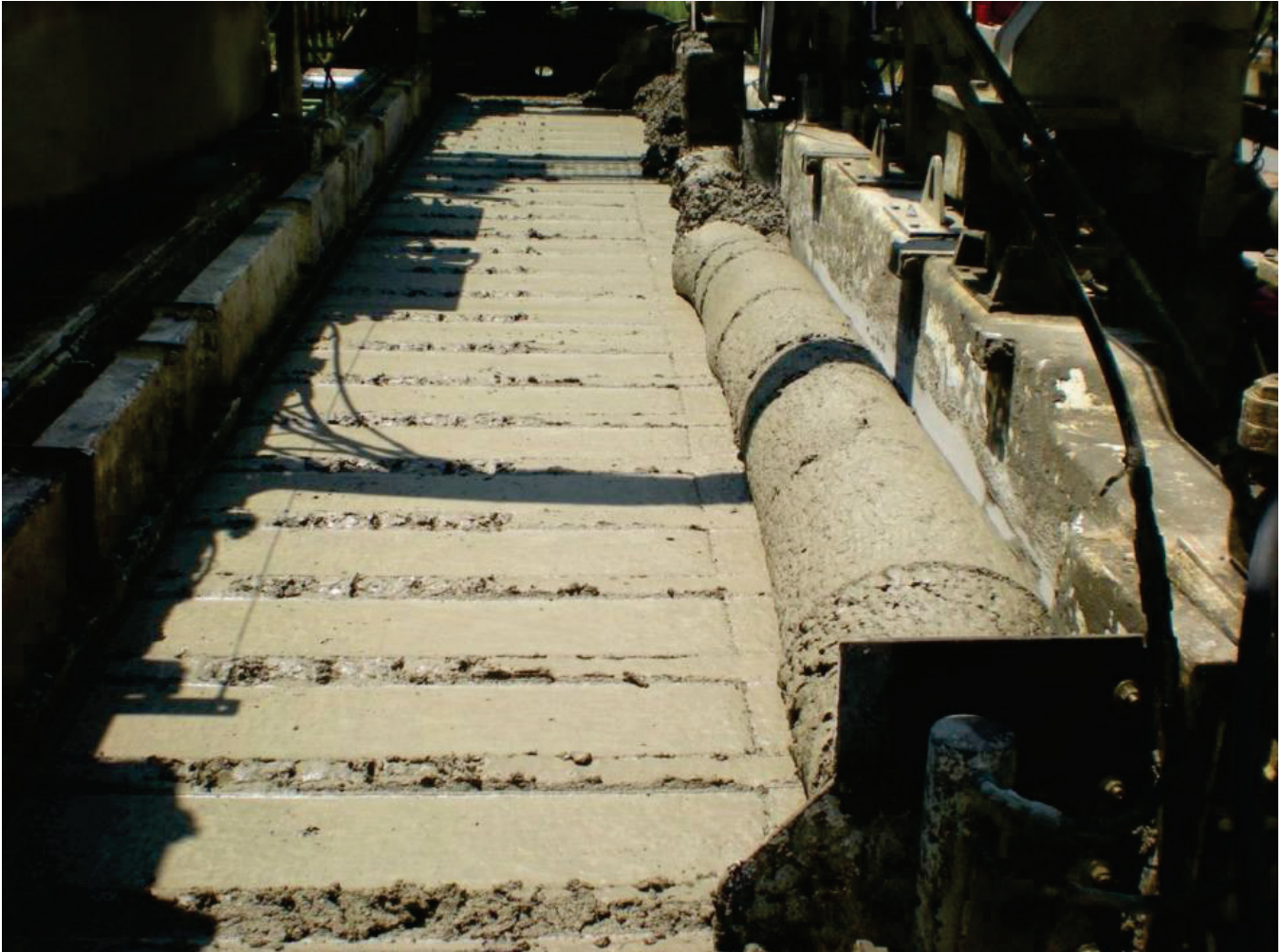
Figure 38 – Automatic Dowel Bar Inserter (DBI)
