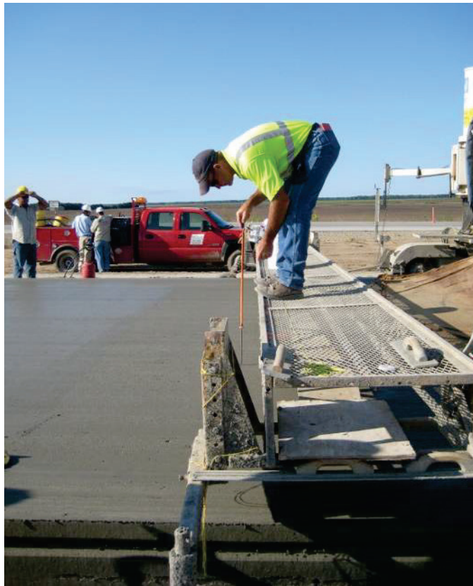
Figure 15 – Thickness Probing Behind the Paver
