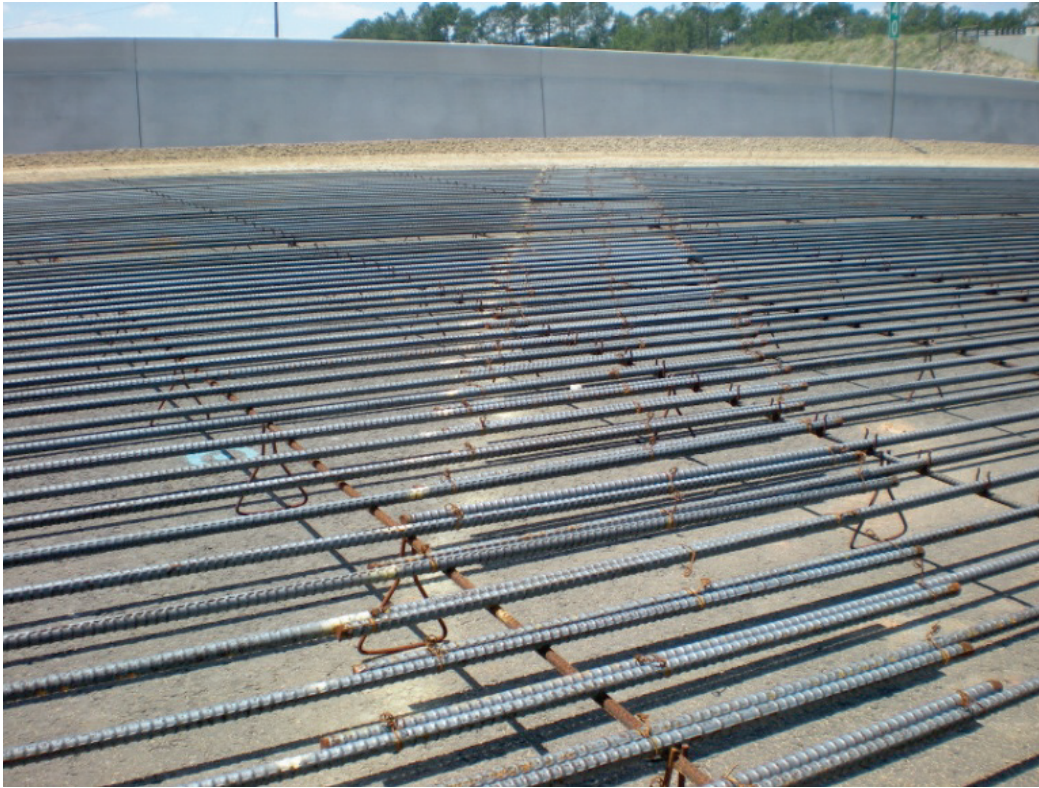
Figure 29 – Staggered Laps for Longitudinal Reinforcing Bars
