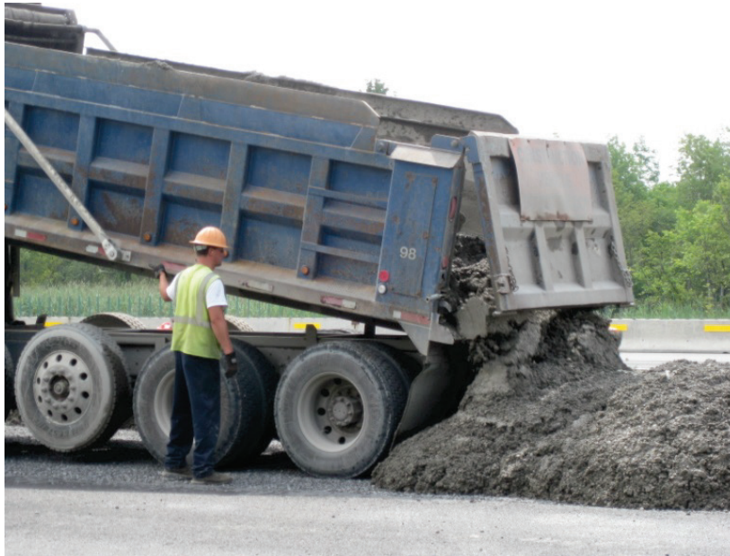
Figure 33 – Transporting Concrete in a Dump Truck
