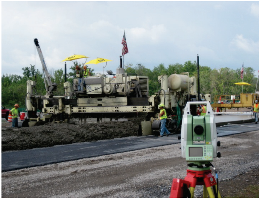
Figure 23 – Stringless Paving Using a Robotic Laser and Radio Communication
