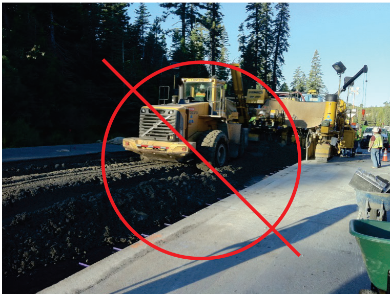
Figure 36 – Adjusting Paver Head with an End Loader
