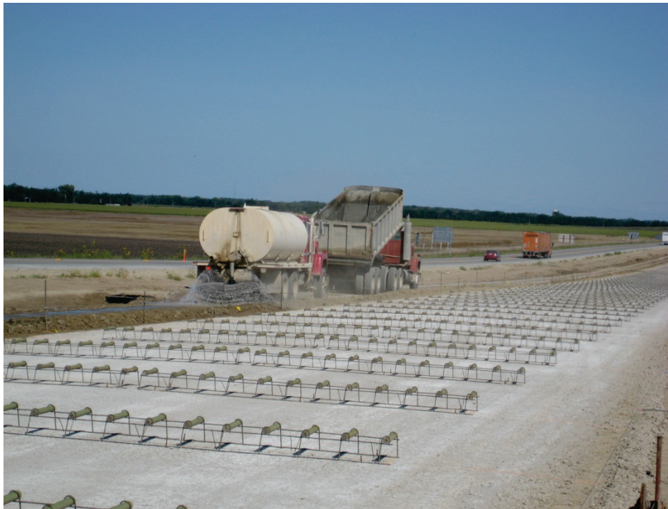
Figure 6 – Jointed Plain Concrete Pavement Before Paving
