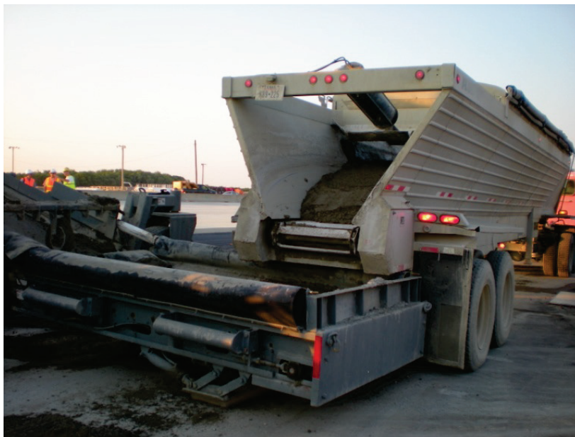
Figure 34 – Transporting Concrete in a Live Bottom Trailer
