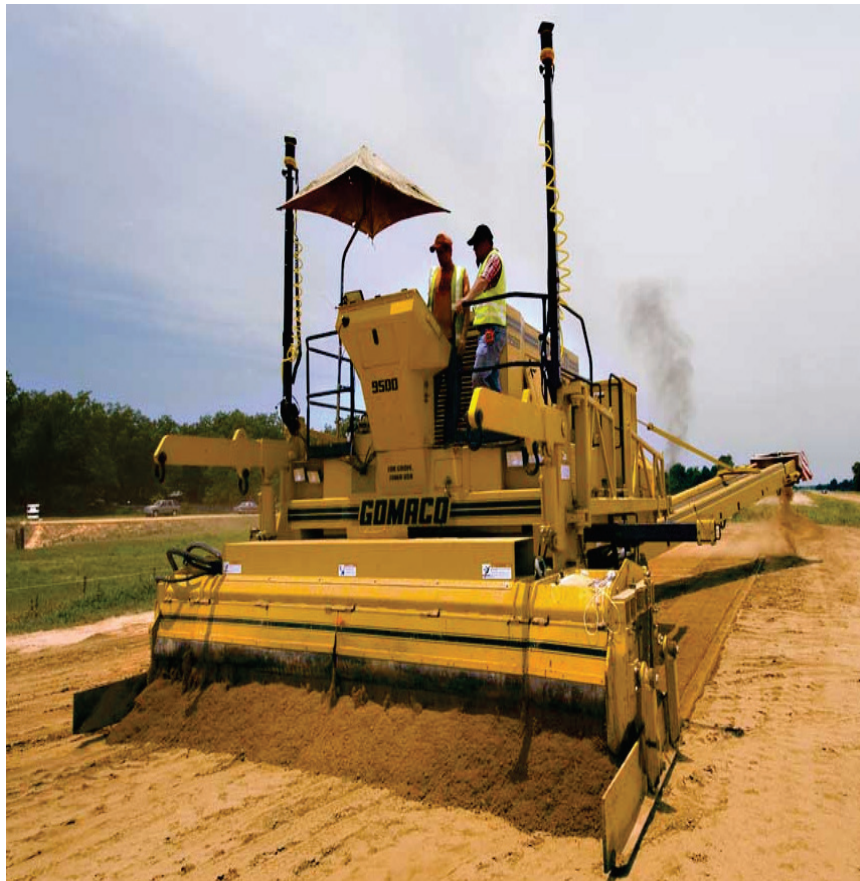
Figure 24 – Fine Grading with a Trimmer
