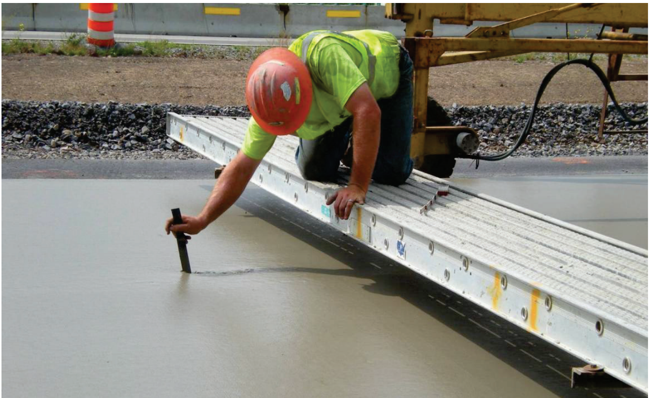
Figure 26 – Probing for Dowel Locations
