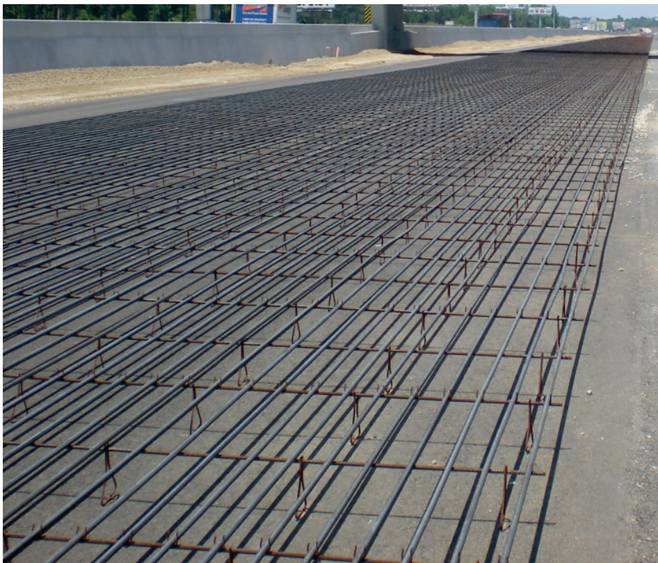
Figure 28 – Properly Supported Reinforcing Steel
