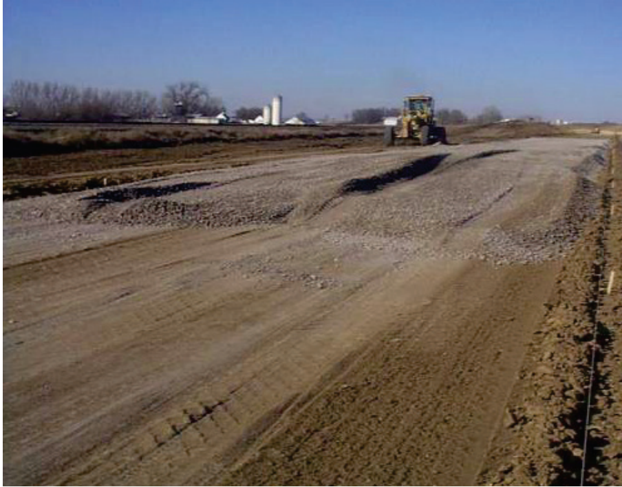
Figure 21 – Visually Inspect Granular Subbase for Segregation
