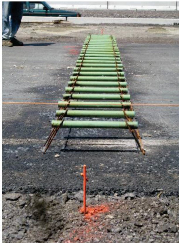
Figure 25 – Positive Marking of Dowel Basket Location for Sawing Joints
