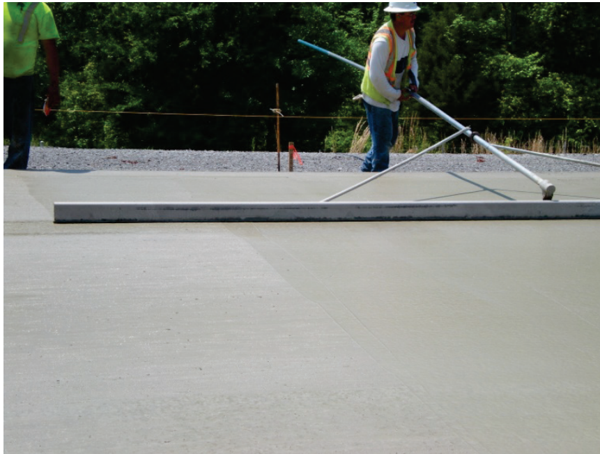
Figure 40 – Using a Straightedge to Identify Dips and Bumps
