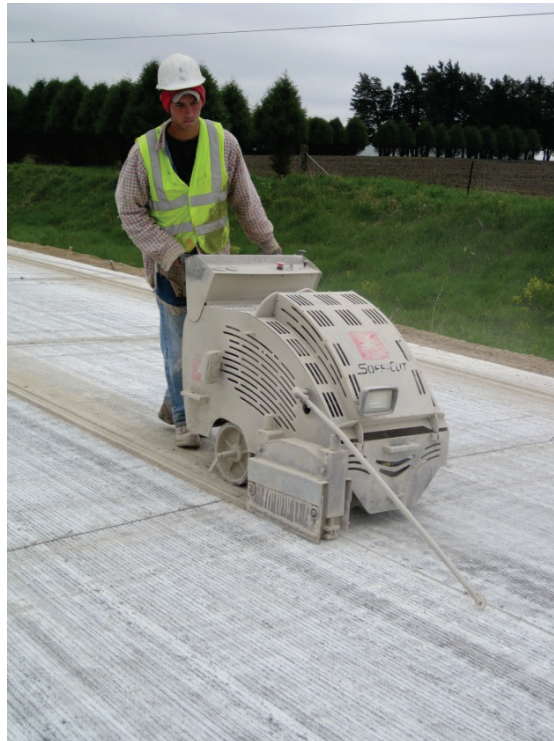
Figure 43 – Sawing Joints Requires Well Maintained Equipment and Experienced Personnel
