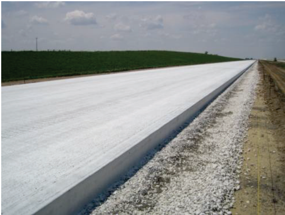
Figure 42 – Complete and Uniform Coverage of Curing Compound
