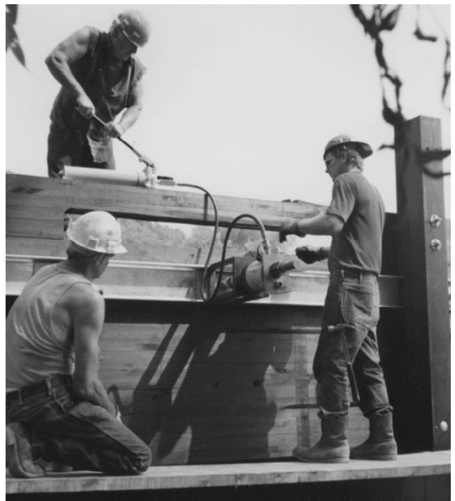
Figure 11—Bar tensioning using a single hydraulic pump and ram.
