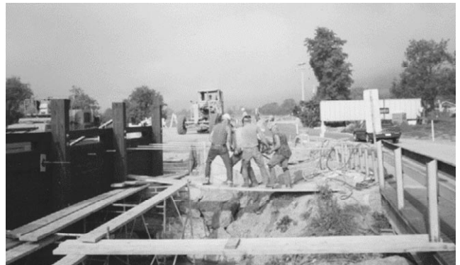
Figure 10—Insertion of tension bars using a jack hammer.
