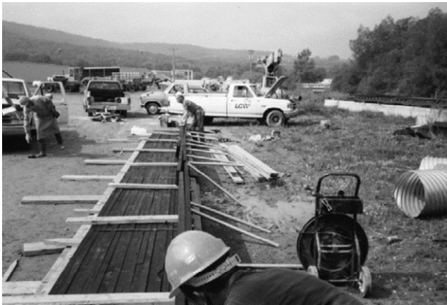
Figure 6—Fabrication of flange assemblies.
