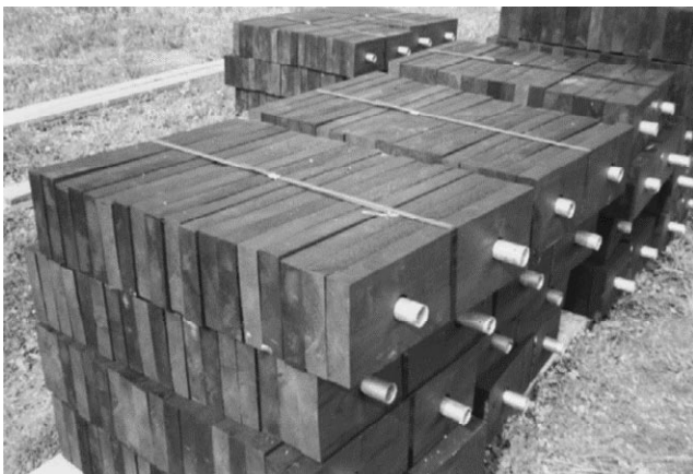
Figure 7—Finished diaphragm assemblies awaiting transport to bridge site.
