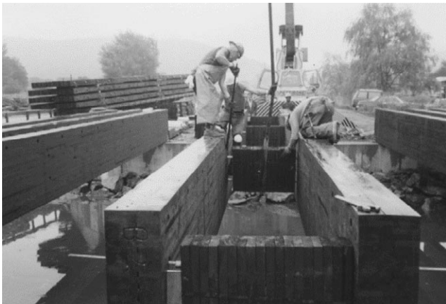
Figure 8—Installation of diaphragm and flange assemblies at bridge site.
