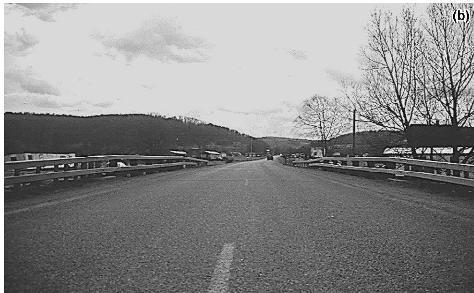
Figure 12—Completed Humphrey bridge: (a) side view, (b) end view.
