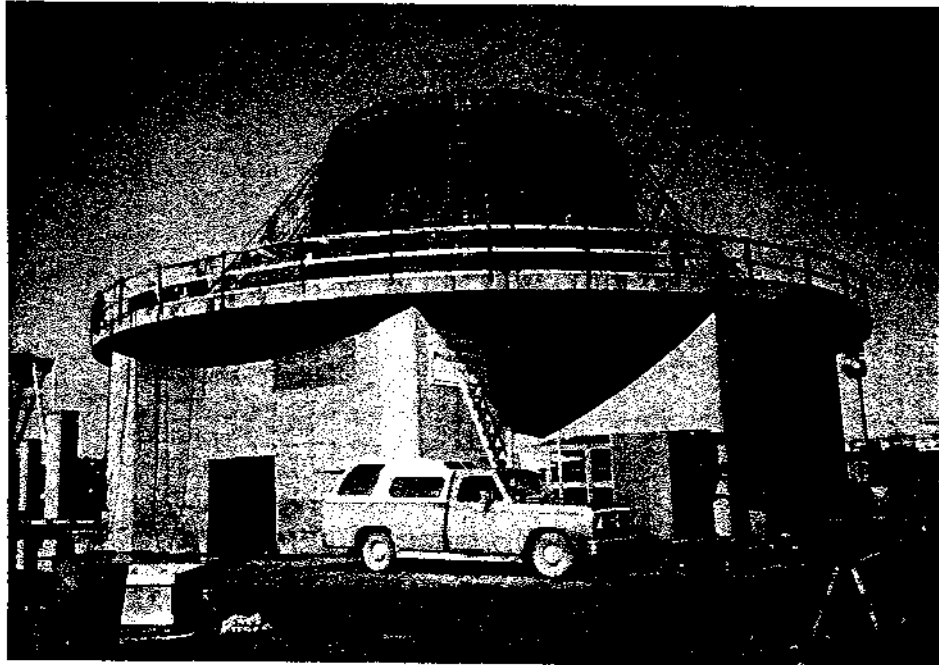
Photo 6: Assembly of Reinforcement for Ice Shield
