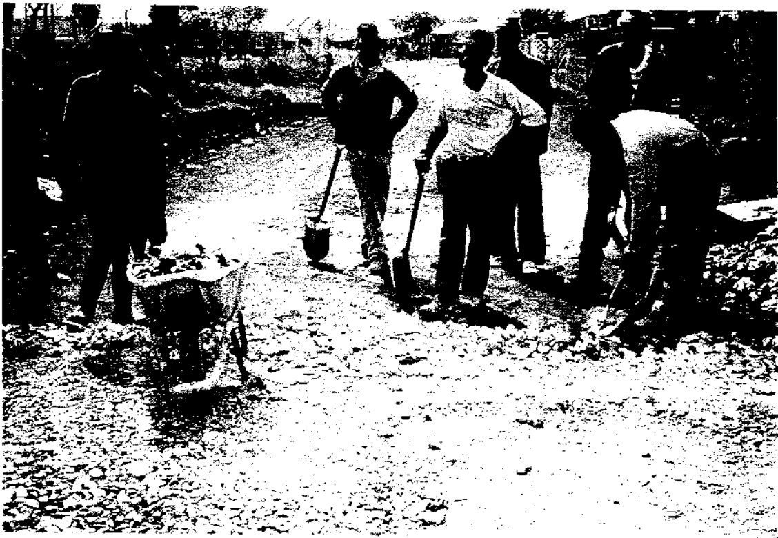
Figure 14. Construction of Water-Bound Macadam Pavement
