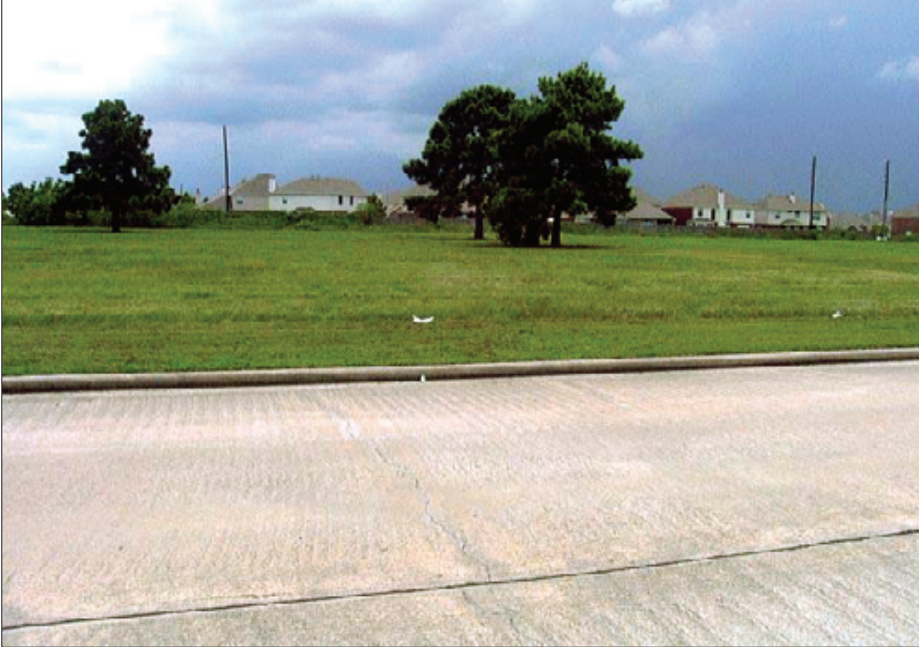
Open space buffer between highway and residential community.
