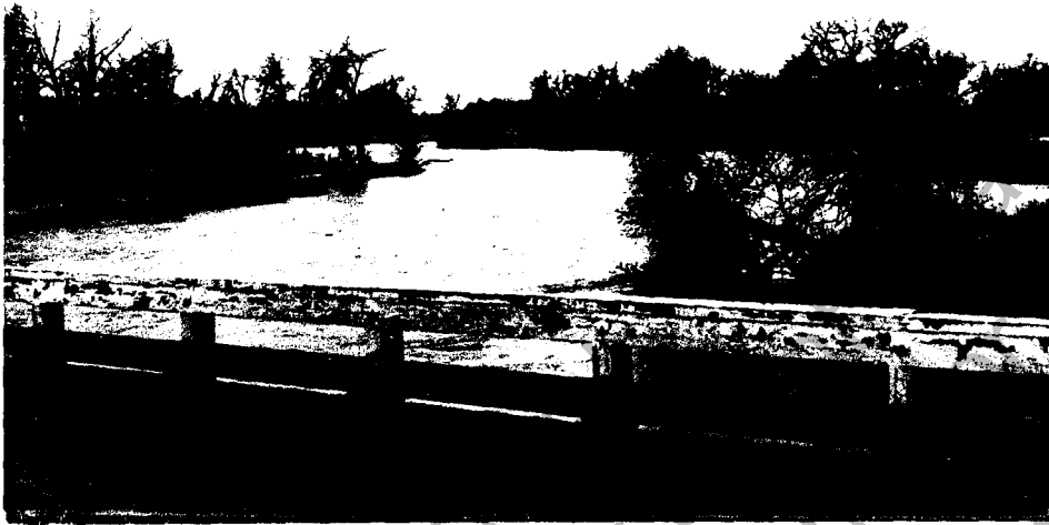
LOOKING UPSTREAM FROM EXISTING BRIDGE
