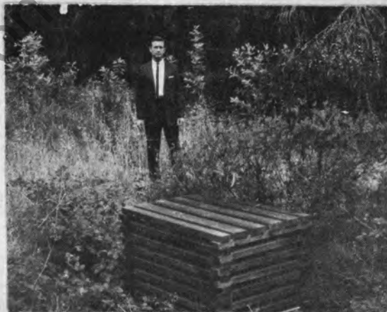
Figure 39. Redwood debris crib with spacing to prevent passage of fine material. Basin had built up 30'.
