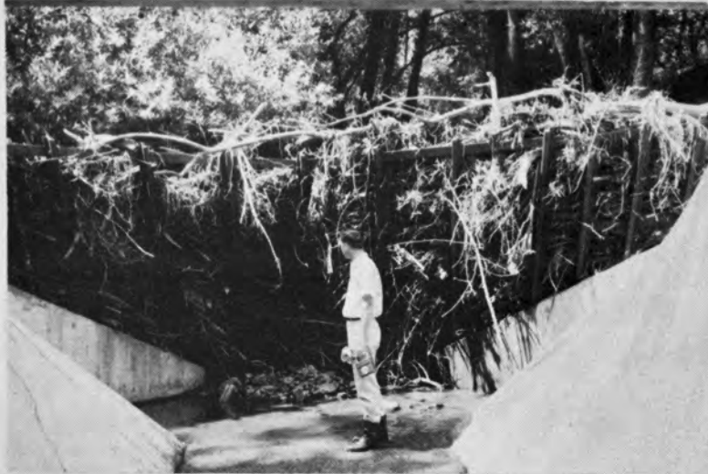
Figure 25. Steel debris rack probably saved the culvert from plugging.
