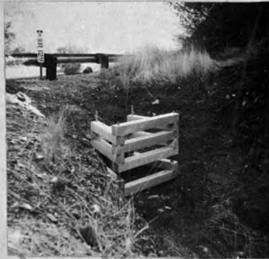
Figure 36. Debris crib of precast concrete sections and metal dowels. Height increased by extending dowels and adding more sections.
