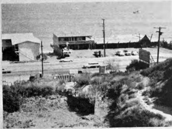
Figure 48. Debris dam and basin in foreground and steel grill debris rack at culvert entrance in background. (See Fig. 49).
