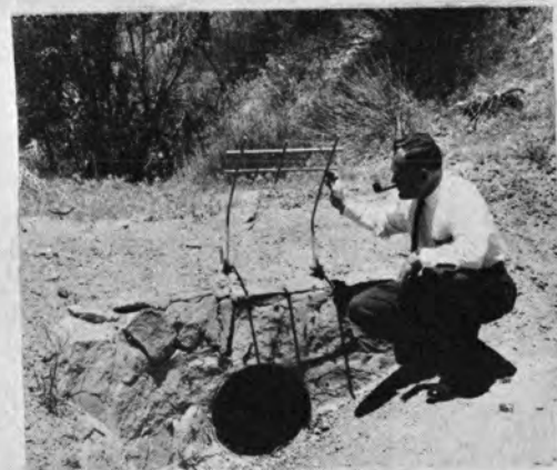
Figure 20. Debris control hinged installation of reinforcing steel at inlet to roadside down-drain.
