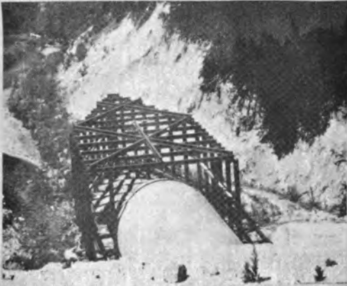
Figure 8. Steel rail debris deflector. Note storage area for debris resulting from culvert projection.
