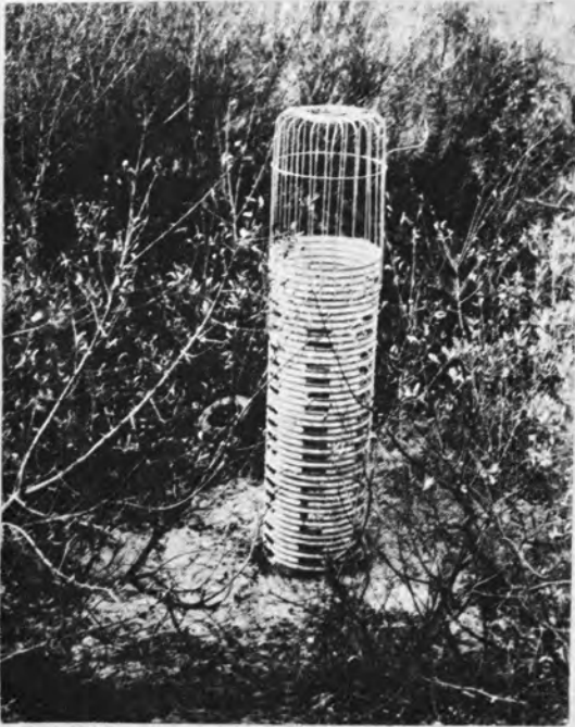
Figure 32. Metal pipe debris riser shows slots for low flows.
