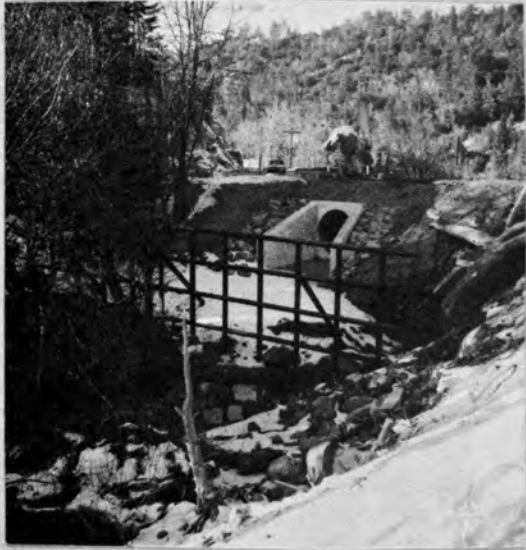
Figure 21. Steel debris rack.
