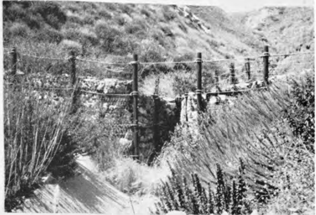
Figure 49. Debris dam of rock and wire shown in Fig. 48.
