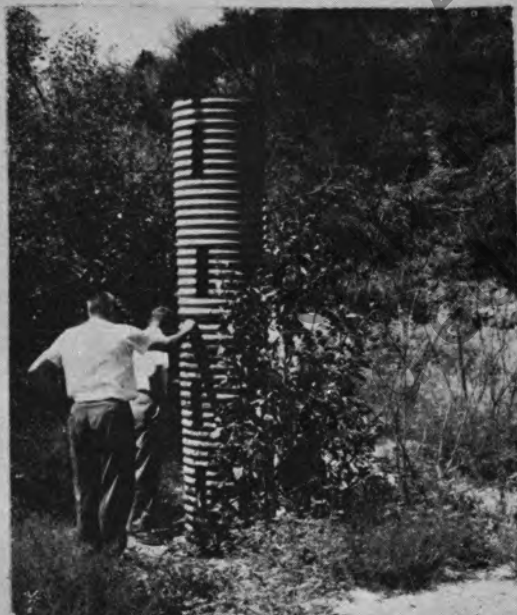
Figure 30. Metal pipe debris riser required little maintenance. Basin had built up 10'.
