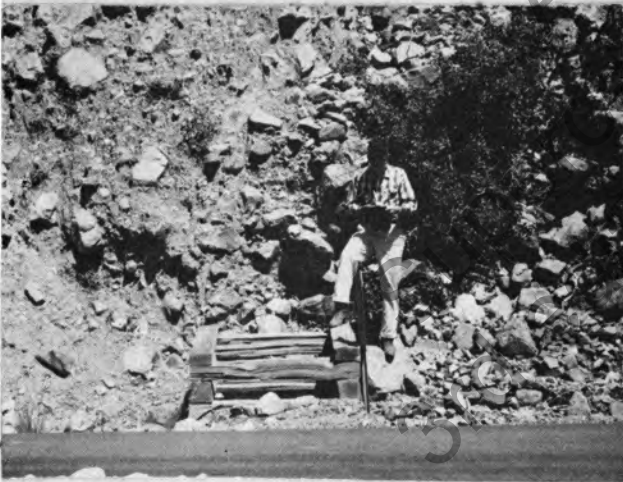
Figure 38. Timber debris crib of inexpensive local materials.
