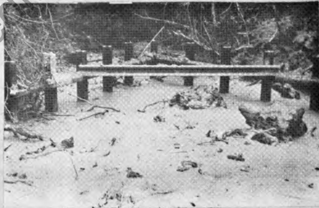
Figure 4. Steel rail debris deflector in area of heavy flowing debris.
