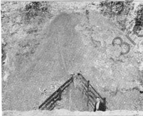
Figure 3. Steel rail debris deflector for fine detritus.
