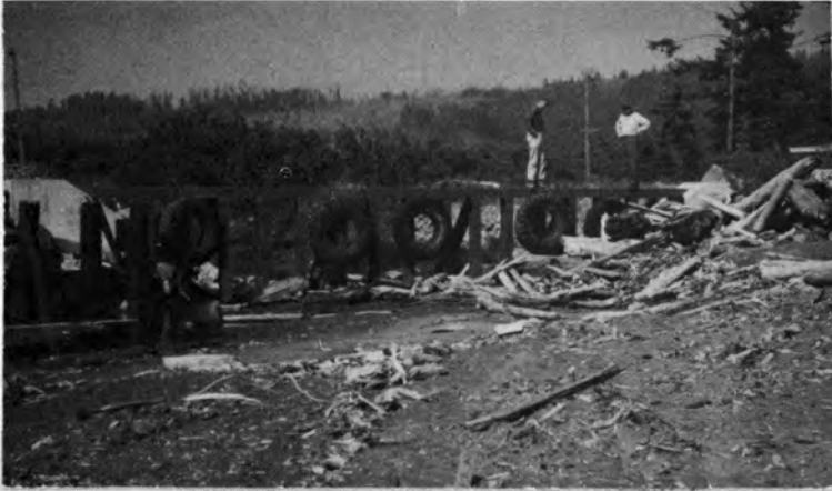
Figure 17. Steel debris rack downstream of culvert on beach. Rubber tires reduce impact of logs.
