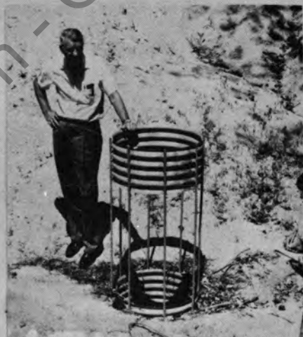
Figure 31. Metal pipe debris riser, in place for 25 years, operated well without vertical extension.
