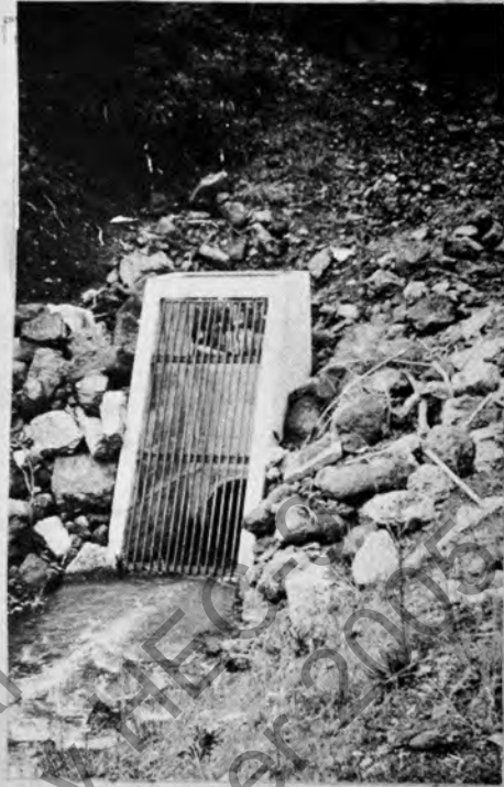
Figure 22. Debris rack used in State of Washington. (See Plate III for design dimensions.)
