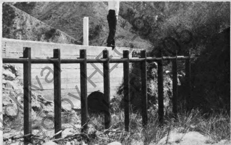
Figure 17. Steel debris rack downstream of culvert on beach. Rubber tires reduce impact of logs.
