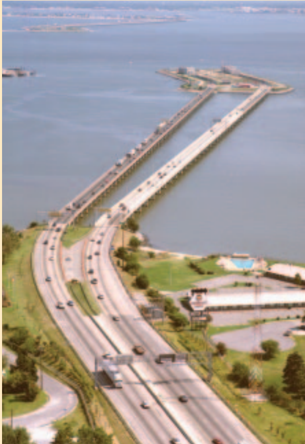
Hampton Roads Harbor Bridge- Tunnel on I-64
