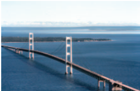
Mackinac Bridge, Mackinaw City
