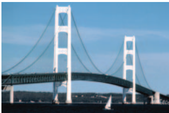
Mackinac Bridge, Mackinaw City
