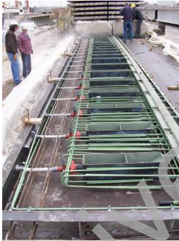
Figure 14. Photo. Joint panel prior to concrete placement, showing post-tensioning pockets, anchors, stirrups and dowels.
