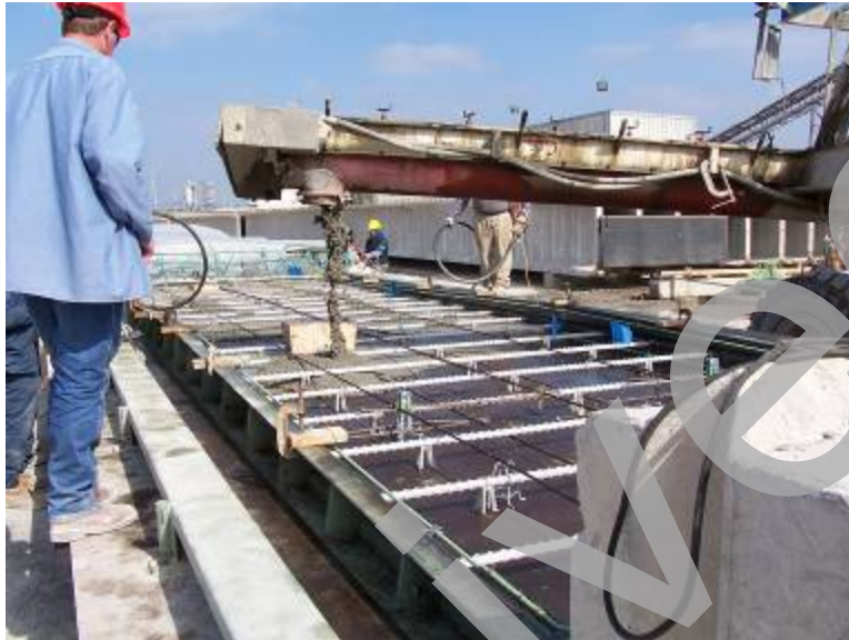
Figure 17. Photo. Concrete placement for a base panel.
