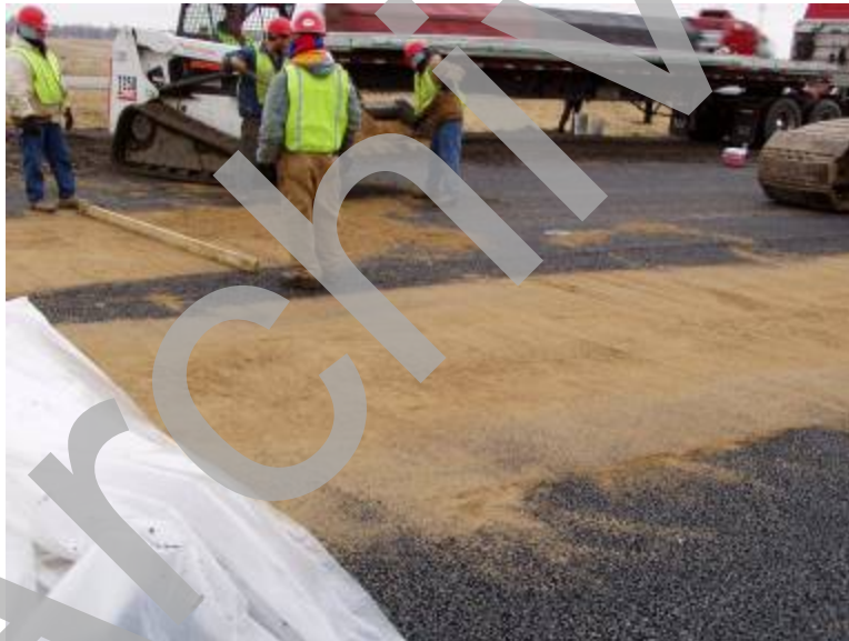
Figure 34. Photo. Sand was used to fill the ruts in the permeable asphalt treated base.
