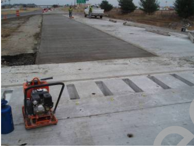
Figure 46. Photo. Adjacent cast-in-place pavement constructed at the end of the PPCP section. (photo from MoDOT)
