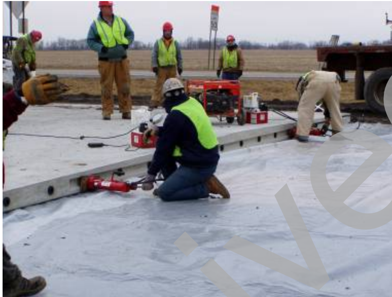
Figure 37. Photo. Temporary post-tensioning was used to close the joints between panels as much as possible during panel installation.
