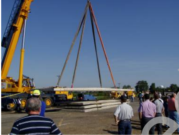
Figure 50. Photo. The workshop participants were able to see a live demonstration of the panel installation process at a MoDOT maintenance yard in Sikeston.
