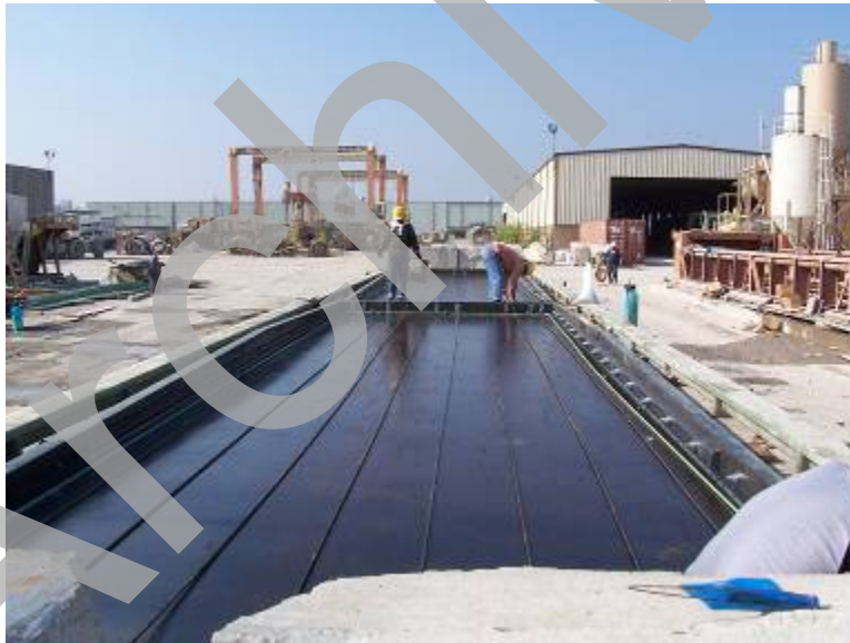
Figure 16. Photo. Precast panel forms during installation of the pretensioning strands.
