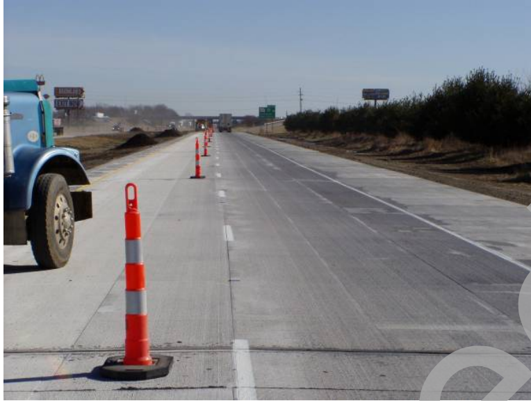
Figure 45. Photo. Final pavement surface after diamond grinding.
