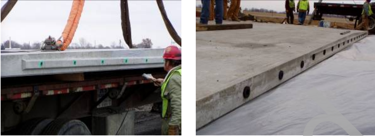
Figure 35. Photo. Epoxy applied to the keyways (left) and installation of the foam gaskets (right).
