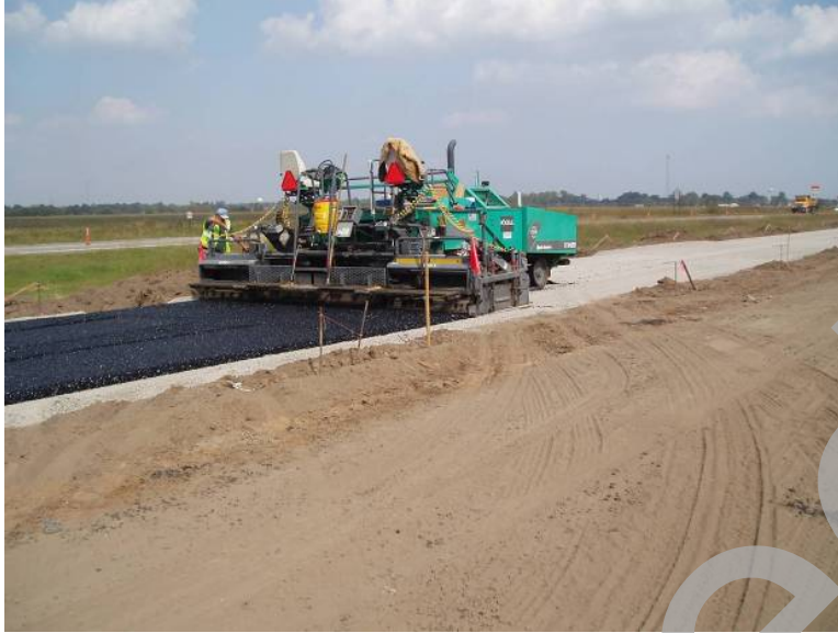
Figure 30. Photo. Construction of the permeable asphalt treated base (photo from MoDOT).
