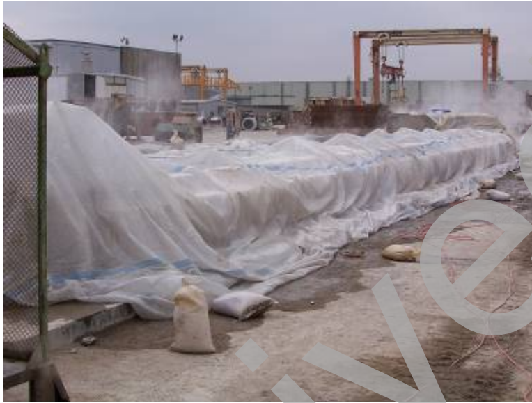
Figure 24. Photo. Casting bed during steam curing operation.
