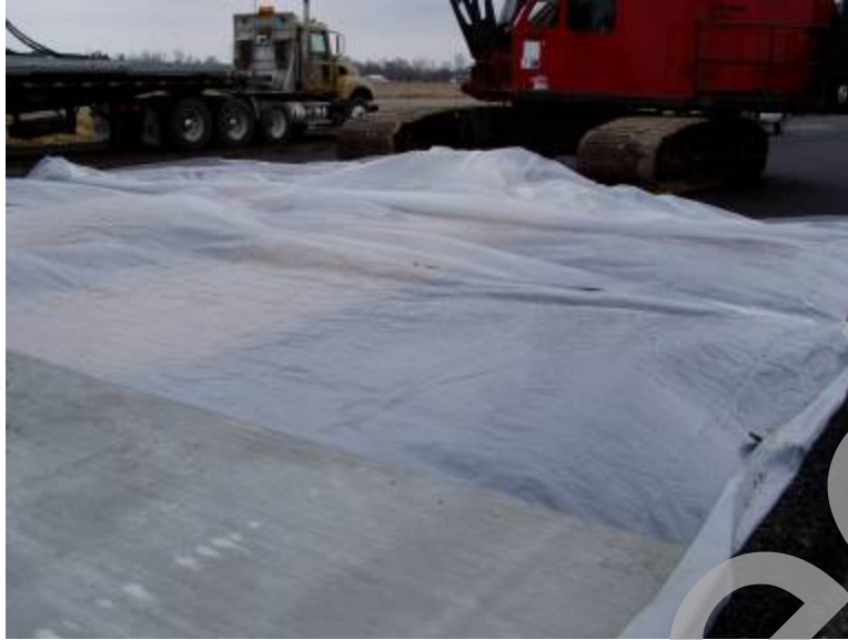
Figure 32. Photo. Polyethylene sheeting rolled out prior to installation of precast panels.
