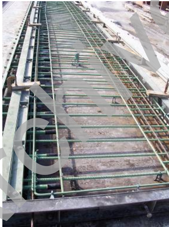
Figure 19. Photo. Reinforcement for the non-post-tensioned half of a joint panel prior to casting.
