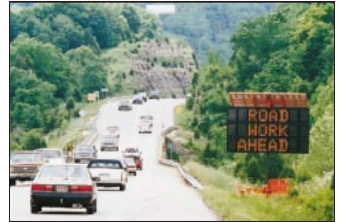
A changeable message sign alerts travelers to anticipate construction delays near Branson.
