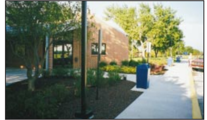
Rest area / I-80 westbound at Kearney
