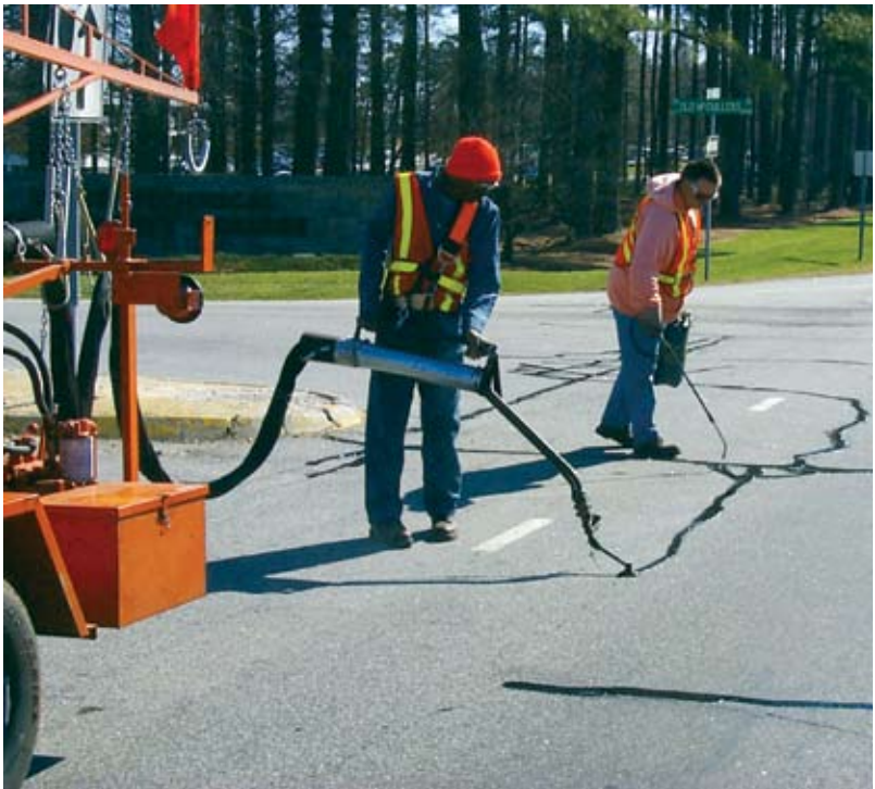
An NCDOT crew crack-sealing a road.
