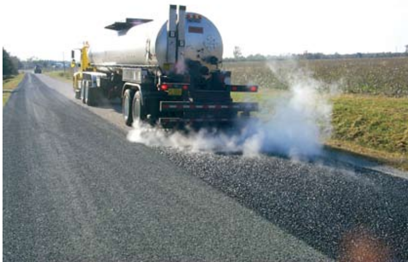
Resurfacing a country road.
