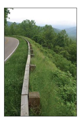
Figure 3.10: Precast Concrete Guardwall, PCG
