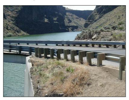
Figure 3.22: W-Beam to Thrie-Beam Transition
