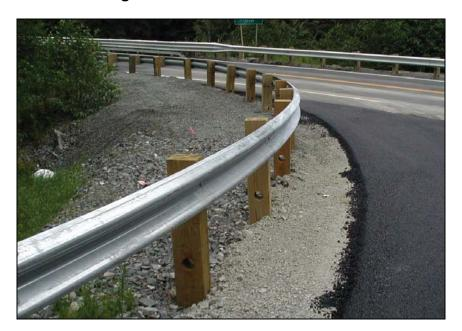
Figure 4.7: Curved Rail Guardrail
