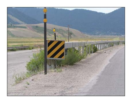
Figure 3.14: W-Beam with MELT
