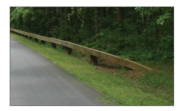
Figure 3.20: Steel-Backed Timber Buried in Backslope
