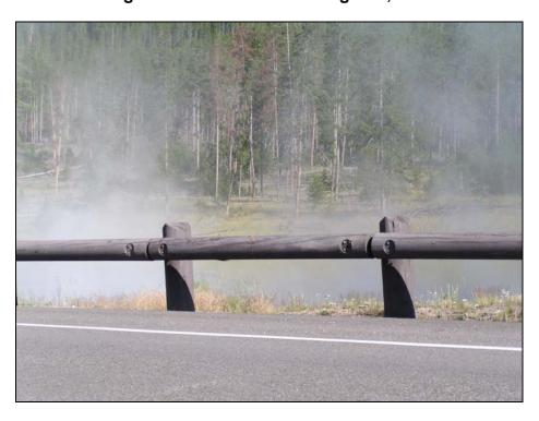
Figure B.8: Steel-Backed Log Rail, SBL
