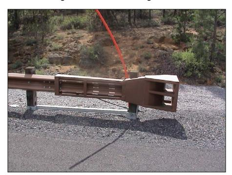
Figure 3.17: W-Beam Tangent End
