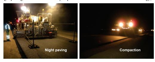
Figure 145. Night paving and HMA compaction.
