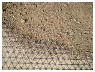
Figure 74. Photographs of TB4 during placement of TX5 geogrid and salvage base layers
