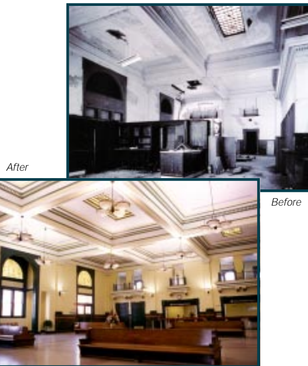
Tampa Union Station in Tampa Bay, FL has been restored to its original use as an active train station and vital transportation hub. (Photo: Florida DOT)
