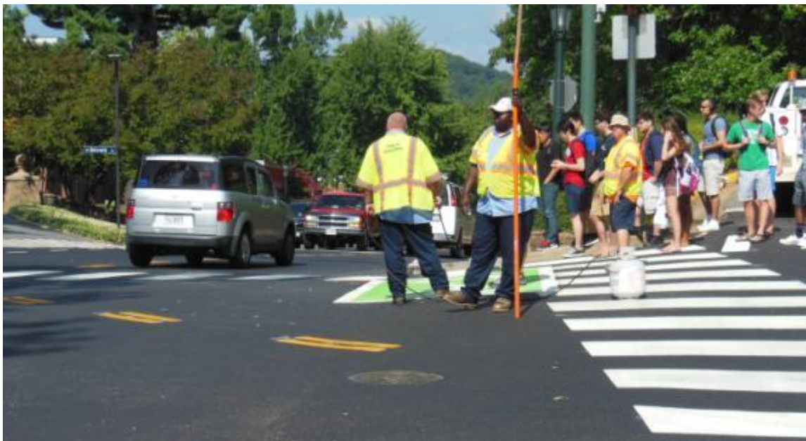
Figure 8. The Two-Stage Turn Box for Westbound University Avenue. This was installed by narrowing / slightly overlapping a crosswalk.
