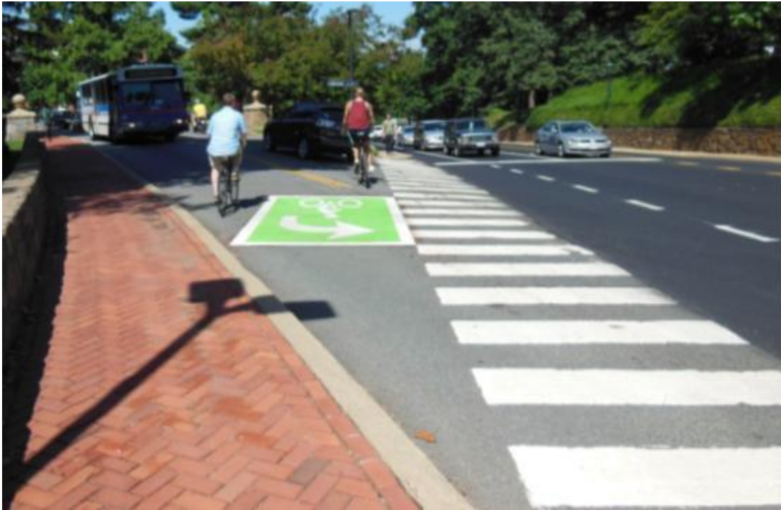
Figure 7. The Two-Stage Turn Box for Eastbound University Avenue. This was installed south of the crosswalk rather than adjacent to its ingress bike lane.
