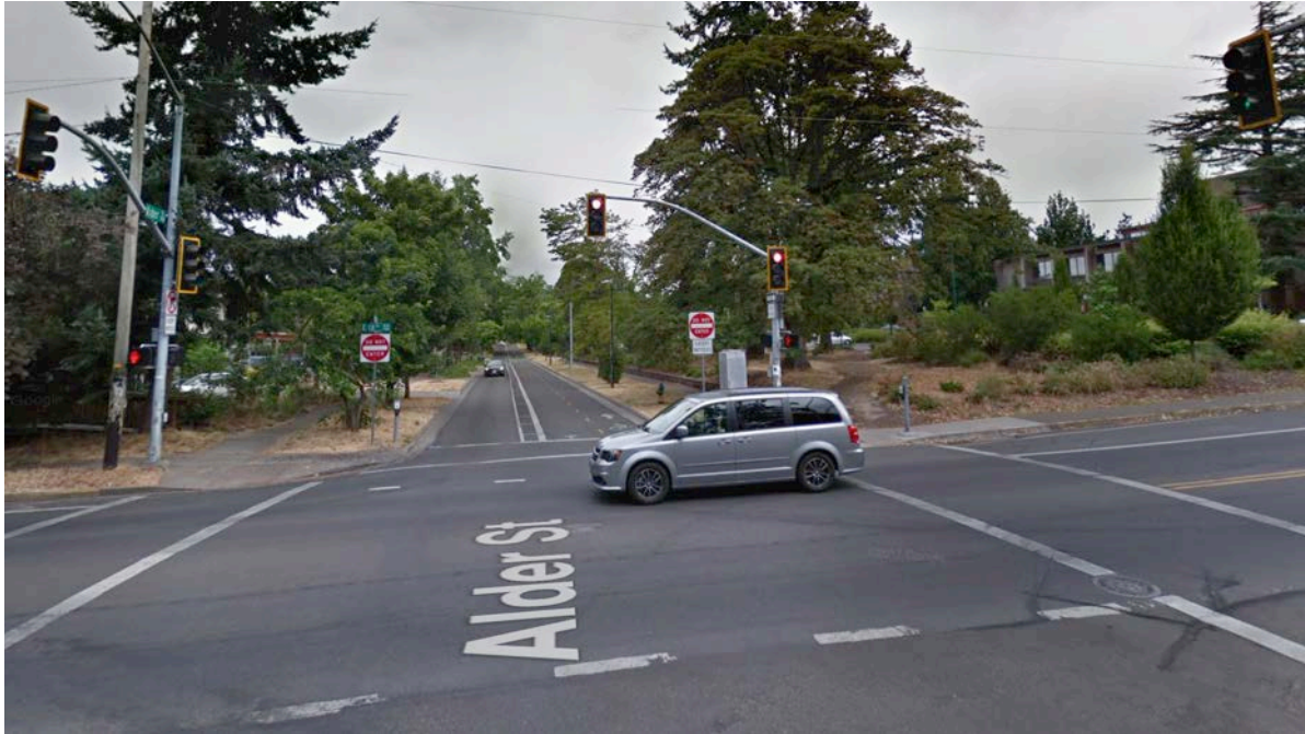
Figure 4: Intersection of Alder and 18th (looking north). Intersection of Alder and 18th (looking north) with bike-only signal (18 th is one-way the other direction at this location). (Source: Google Street View, August 2017 (accessed 7/4/2018)).
