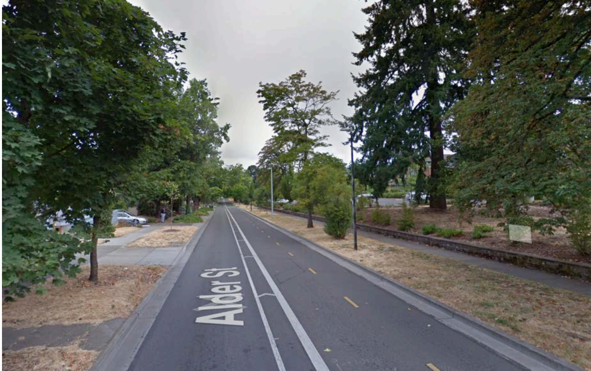
Figure 3: Alder Street section adjacent to University of Oregon. Alder St., equal allocation to bicycle travel (on right) as motorized vehicle travel (on left). (Source: Google Street View, August 2017 (accessed 7/4/2018)).
