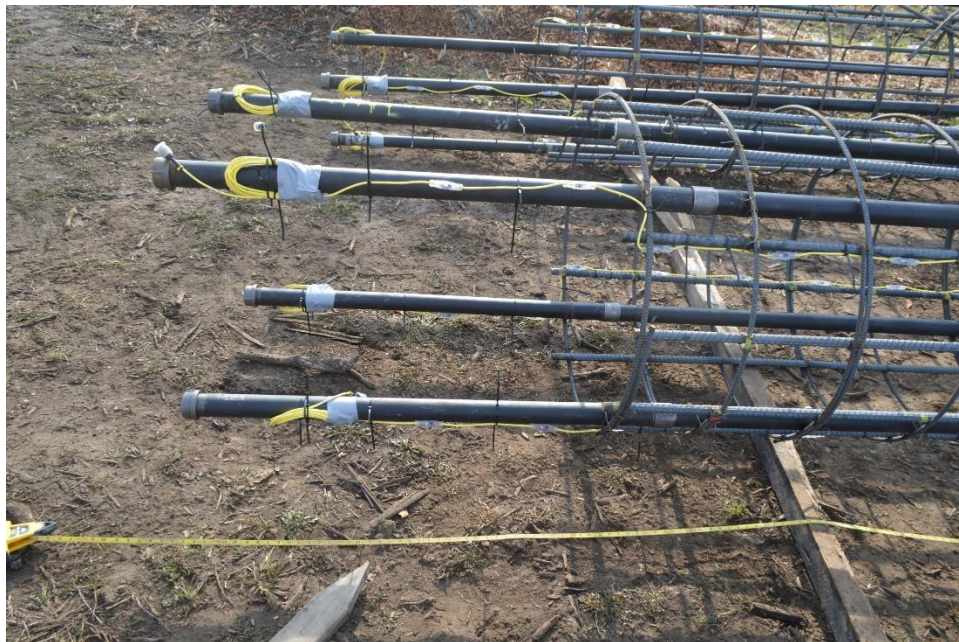
Figure 37: TIP wires exiting the top of the reinforcing cages. Two sensors were above the top of the shaft to measure ambient temperature.
