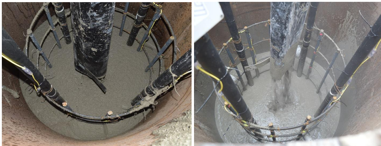
Figure 34: Concrete placement near the top of shaft: (a) normal concrete in Control Shaft and (b) weak concrete for Defect 6 in Test Shaft 1.
