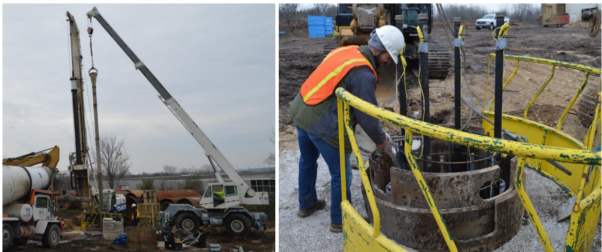
Figure 33: To simulate a tremie breach for Defect 8: (a) the tremie was removed from the shaft prior to (b) placing 30 gallons of water and 70 lbs of sand into the shaft (to simulate a tremie breach in a wet shaft).
