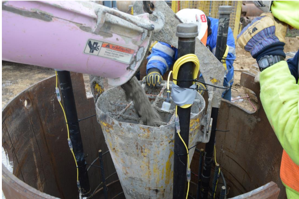
Figure 29: Placement of concrete from the concrete truck to the tremie pipe.
