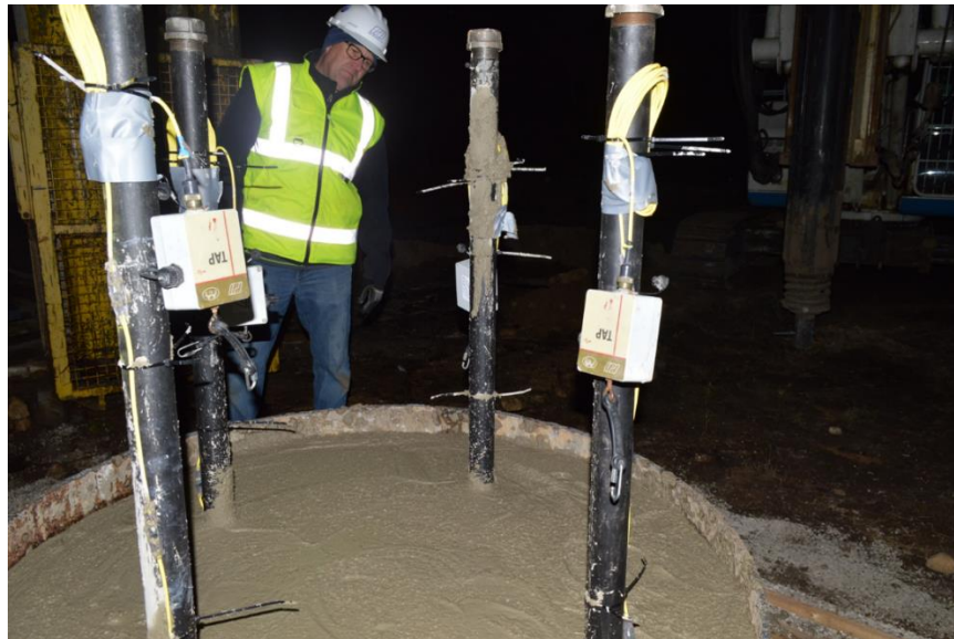
Figure 38: One TAP box was connected to each TIP wire to collect and store temperature data.
