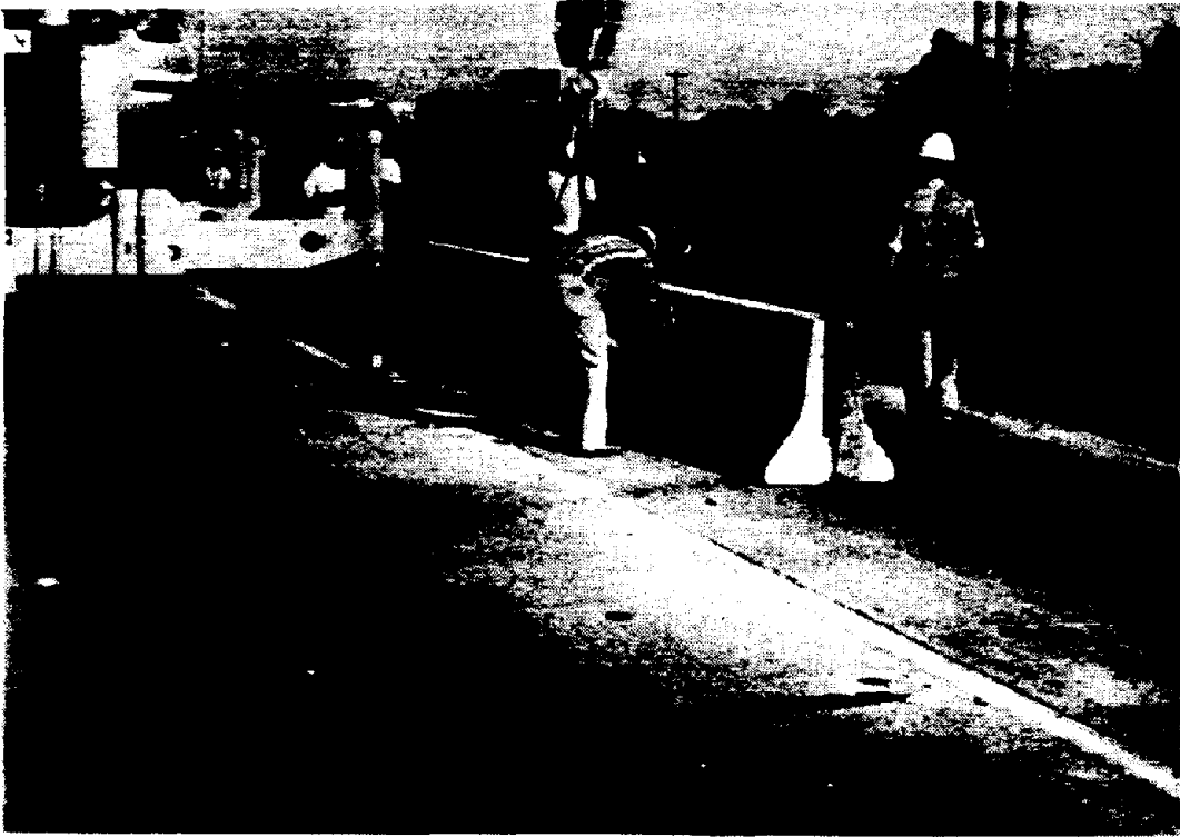
Figure 108. Method 1--Removing Hoisting Rods after Placement.
