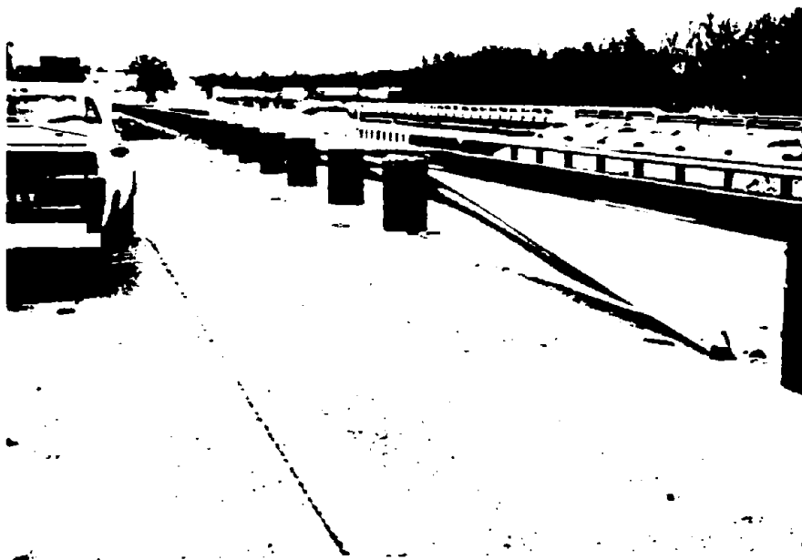
Figure 71. Turned-Down End Treatment on a Barrel/W-Section Barrier.
