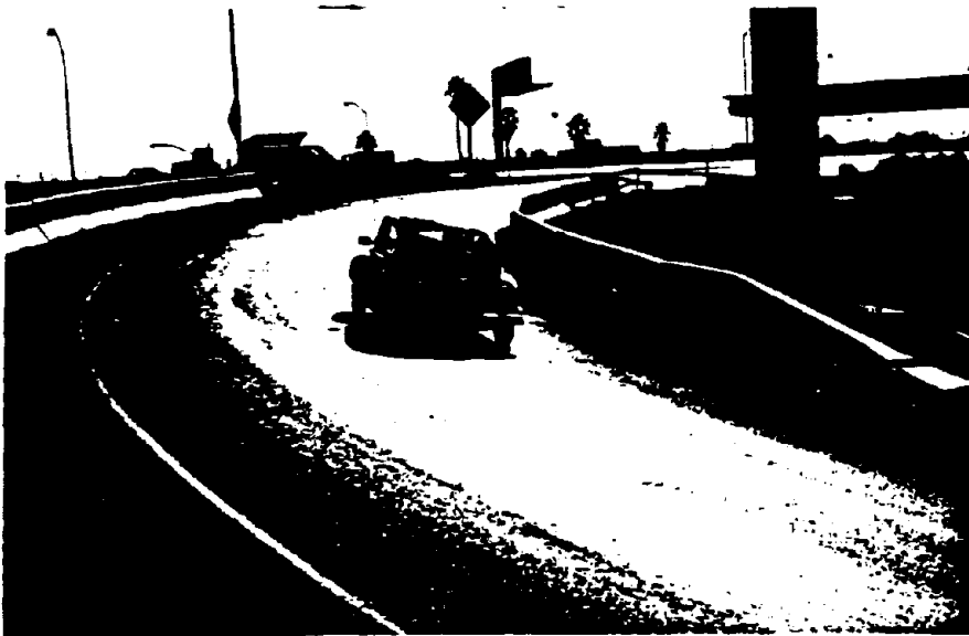
Figure 64. Wedge End Treatment.
