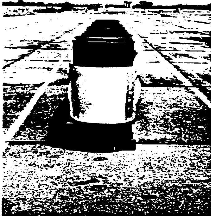
Figure 69. Experimental Barrel/W-Section Crash Cushion.
