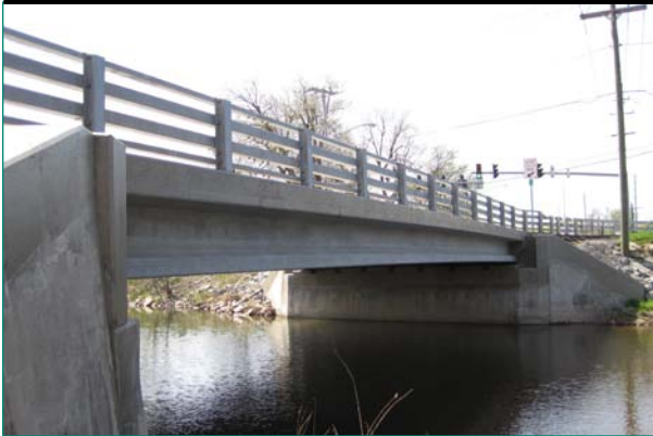
Figure 1. Route 31 bridge in Lyons, NY.
