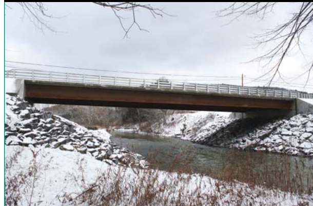
Figure 2. Route 23 bridge in Oneonta, NY.
