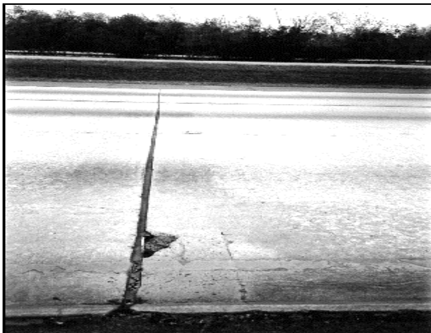
Figure 9.22 Photograph of Poorly Performing Joint Shown in Displacement Profiles in Figure 9.21
