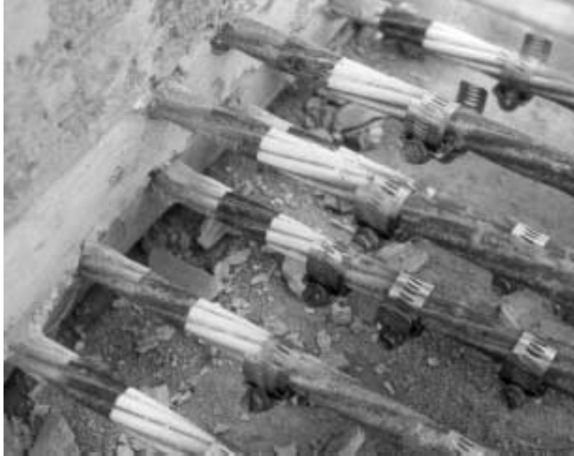
Figure 6.3: Strands Painted to Provide References for Draw-In Measurements
