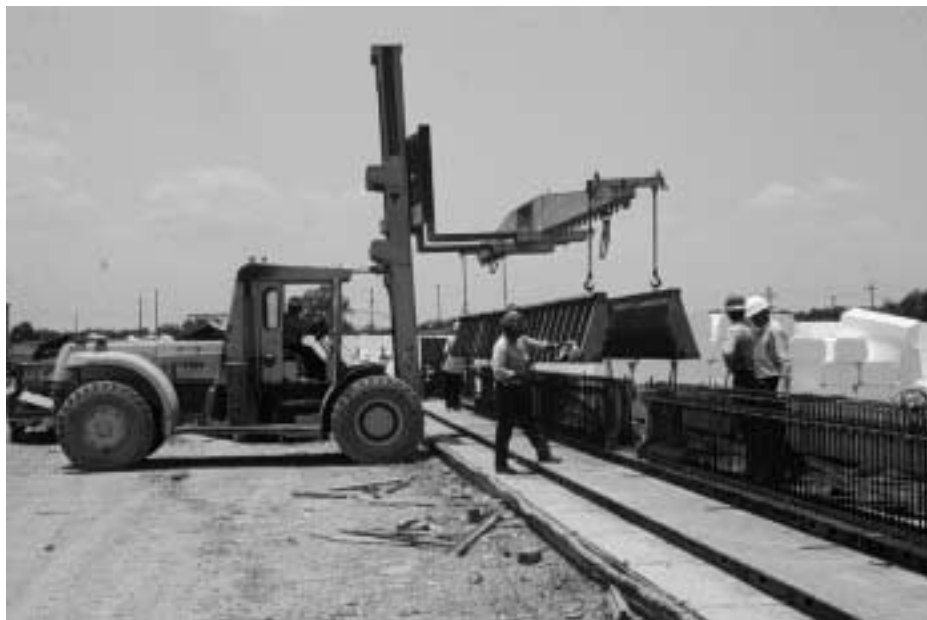
Figure 3.15: Placement of Side Forms
