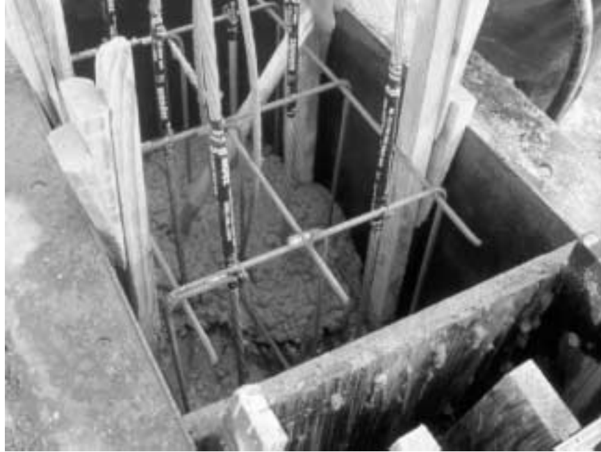
Figure 4.2: Pull-out Test Block at Onset of Casting
