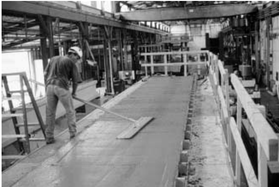
Figure 3.21: Bull-Floating Surface of Slab after Casting
