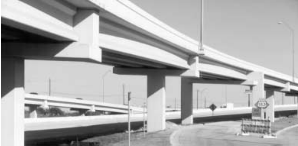
Figure 1.1: Highway Bridge Featuring Precast, Prestensioned I-Beam Superstructure
