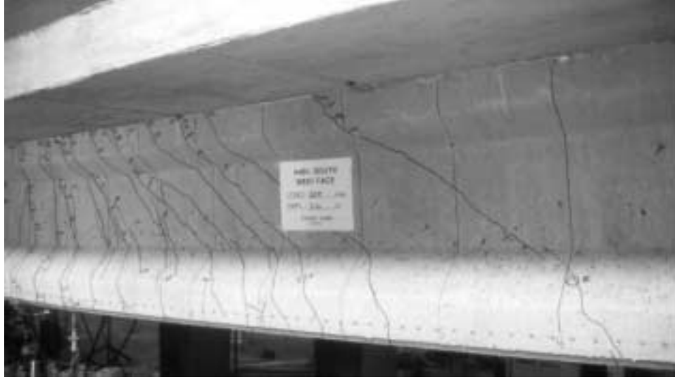
Figure 7.26: Test H4B-D-62—Extent of Cracking at End of Test
