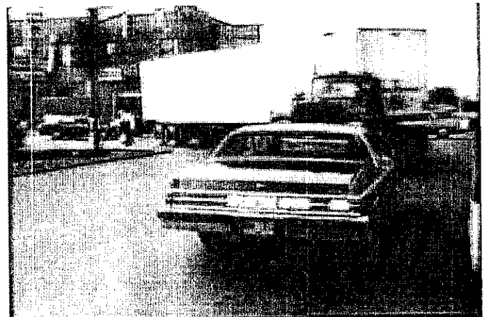
Another aspect is the hazard created by the left turning bay: The car here will have to back up
