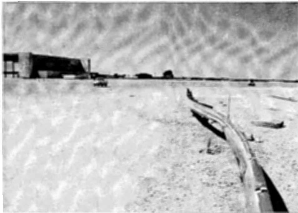
Figure 14. Long-Span Guardrail System Damage, Test OLS-3 (Design No. 3)
