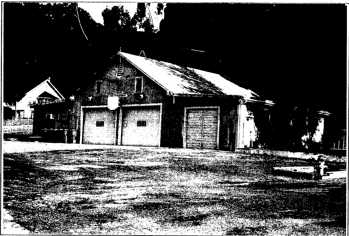
Photograph E.1-5: Firehouse (Building 13)
