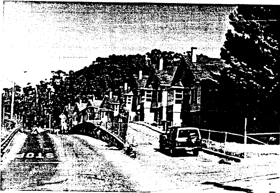
Figure 12: Photograph of Cottages
