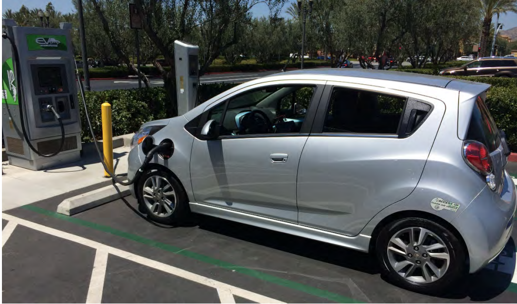
Figure 14 - Public charging station in Irvine, CA.
