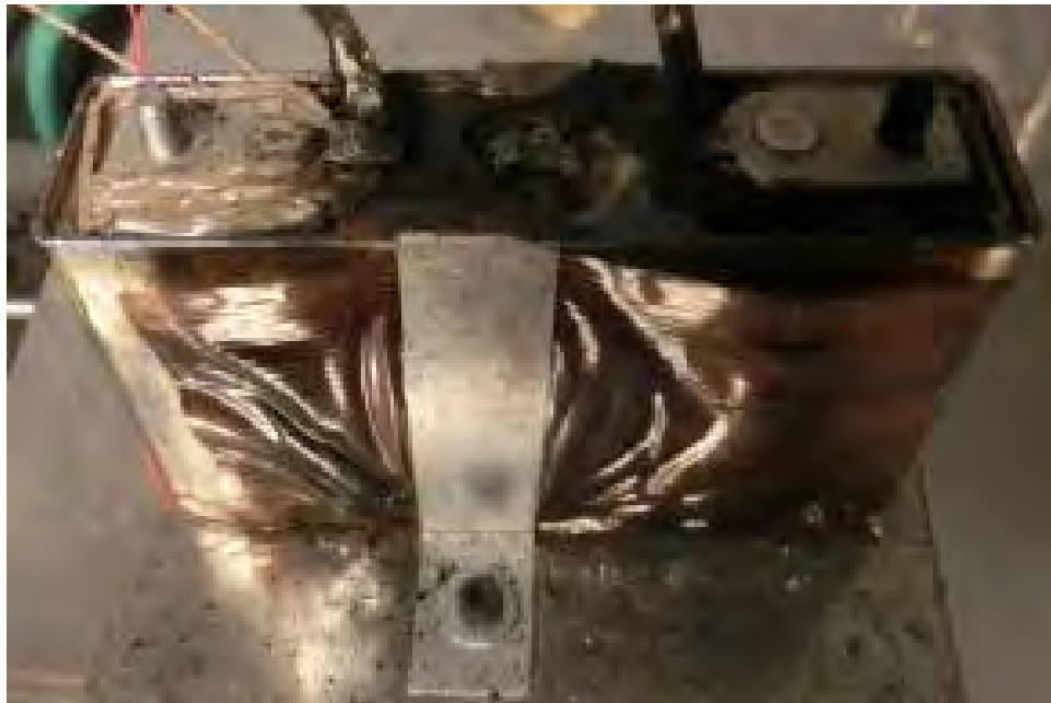
Figure 42 - Prismatic cell after thermal runaway.
