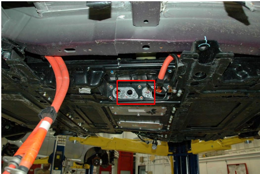
Figure 16 - Manufacturer B vehicle; the high voltage cable pass through (red box) into the RESS (the high voltage cables have been disconnected and are hanging on the left).
