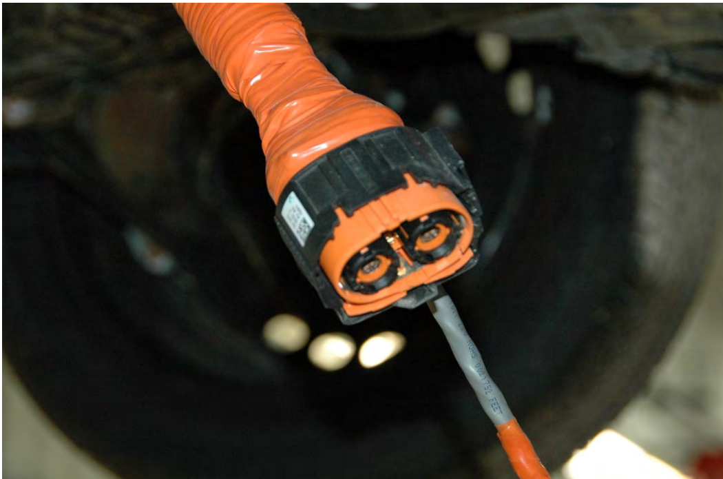
Figure 19 - Manufacturer C vehicle; high voltage cable connector.
