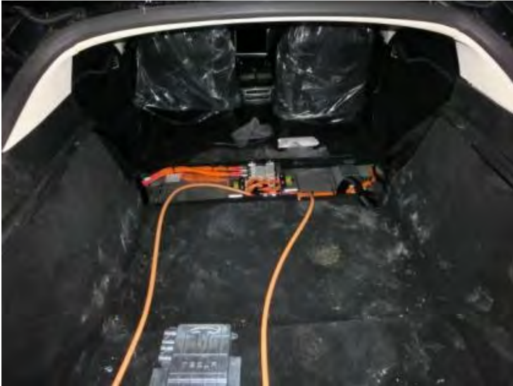
Figure 37 - The location of the exposed DC junction box in the Manufacturer A vehicle. The light orange leads connect to the DC link. Note that the vehicle rear seats have been removed. The junction box cover can be seen on the lower left.
