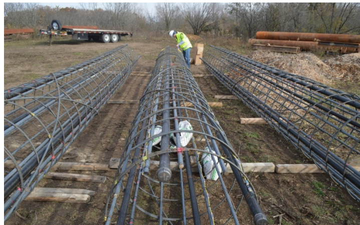
Reinforcing cages prepped with sensors and sandbags
