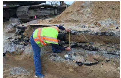
(i) Pavement layer thickness at STH 36
