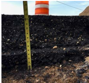
(g) Exposed aggregate base at STH 142E Burlington
