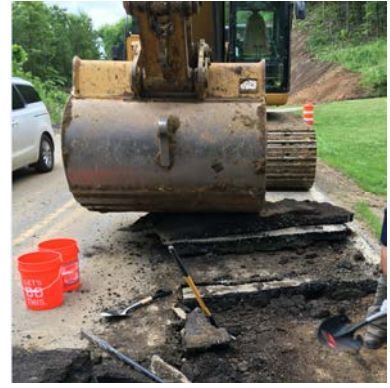
(c) Pavement surface removal at STH 162
