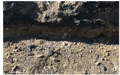
(f) Exposed aggregate base layer at Edgerton Ave
