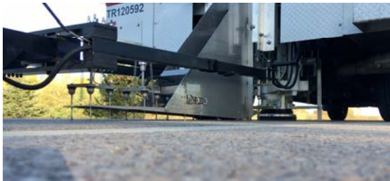
(c) FWD plate and sensors on pavement surface
