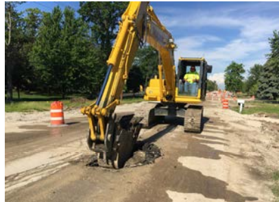
(e) Pavement surface removal at Edgerton Ave
