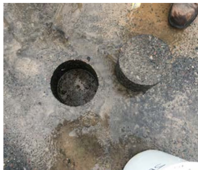
(h) Coring at STH Forest County
