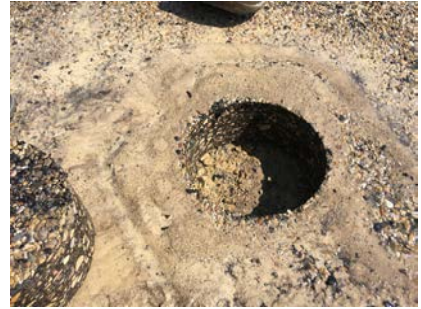
(c) Exposed base aggregate at STH 59
