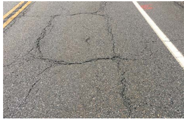
(f) Fatigue and block cracking
