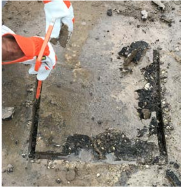
(a) Saw-cutting of pavement surface at STH 33 MR
