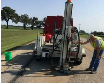
(a) WisDOT coring rig at STH 59
