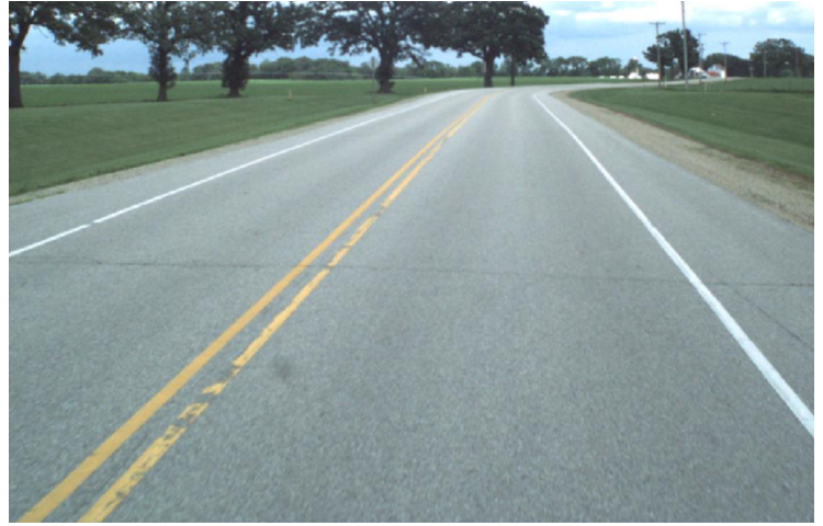
b) Pavement surface distresses
