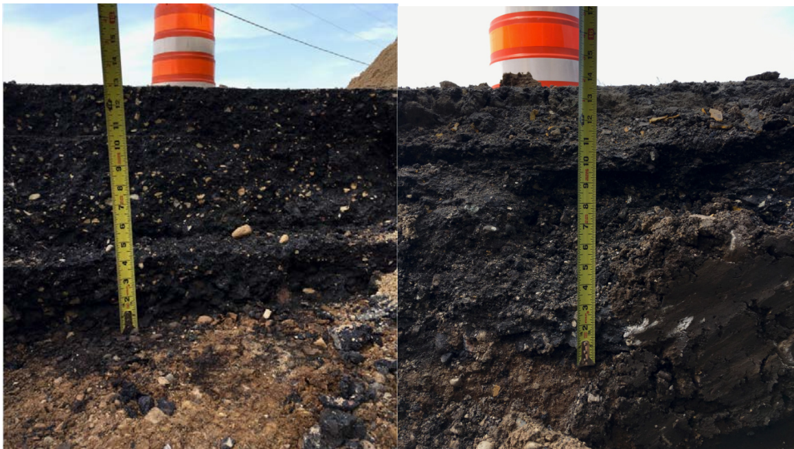
(b) Measured thickness of the excavated pavement layers
