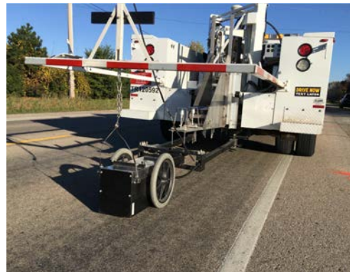
(f) The 900 MHz GPR antenna
