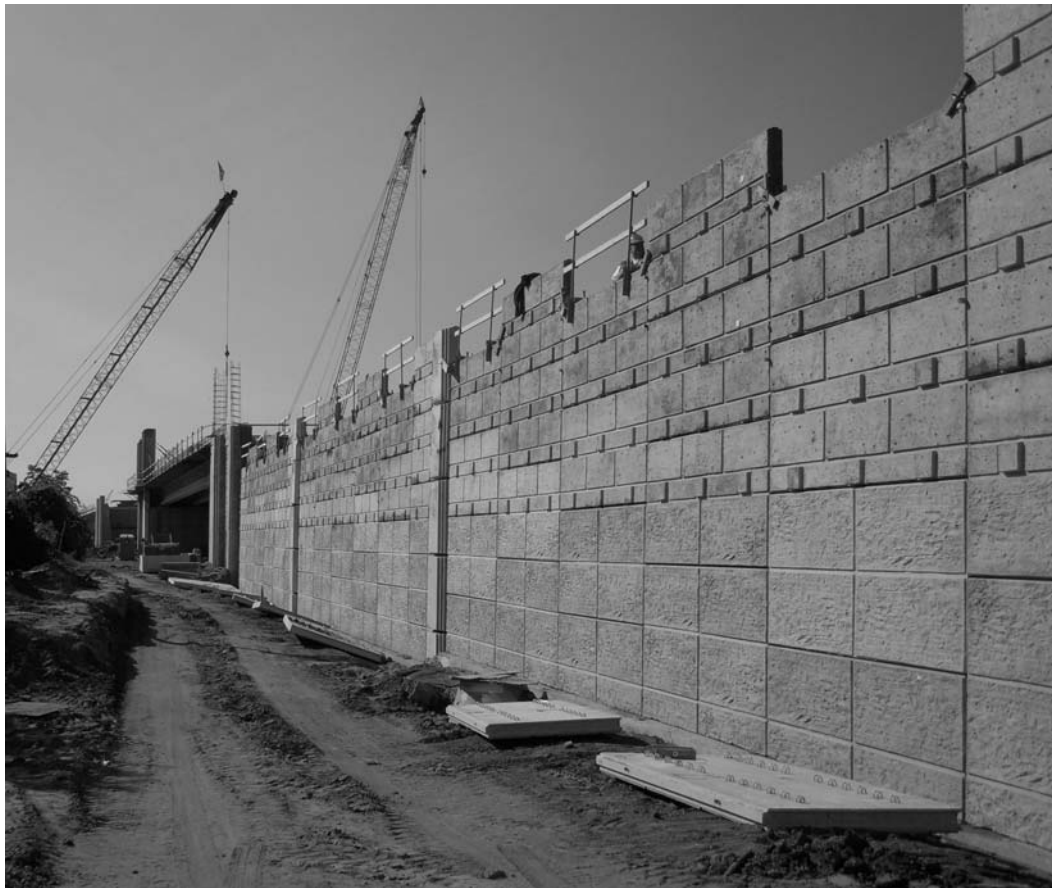
Figure 2-17. MSE wall construction on Mn/DOT Crosstown Project, 2008.
