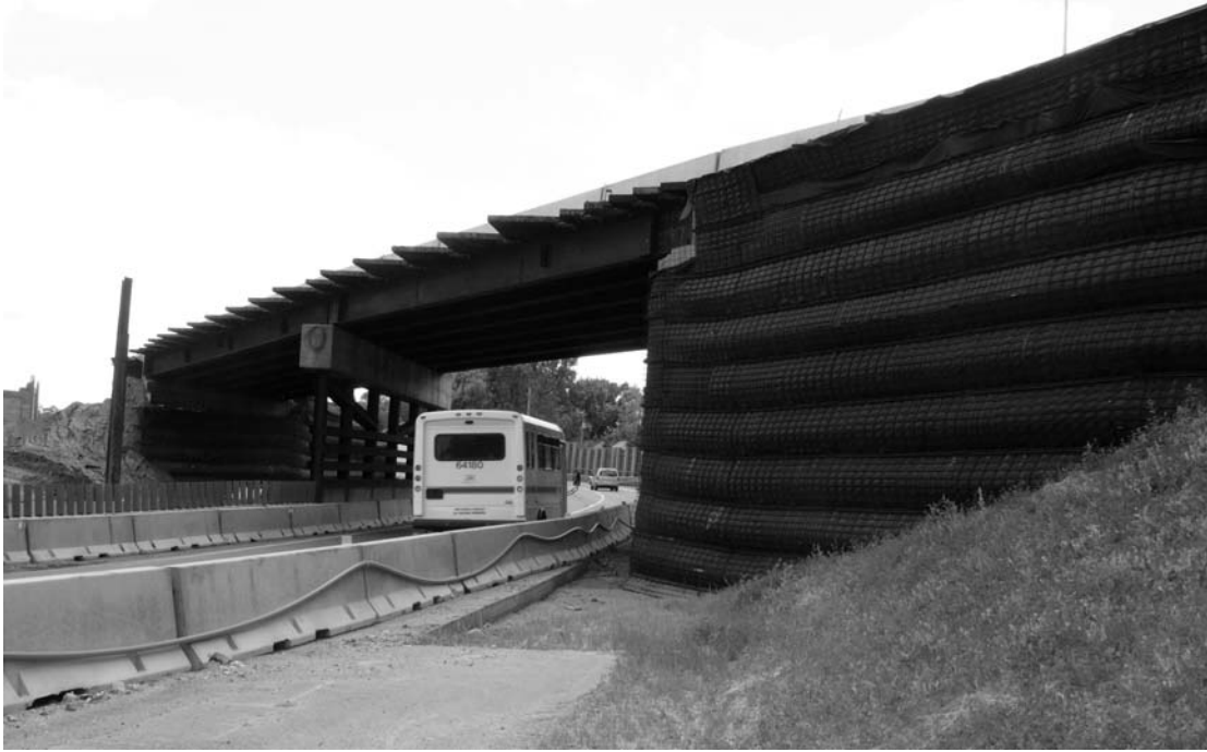
Figure 2-2. MSE walls to support temporary bridge abutment and roadway embankment.
