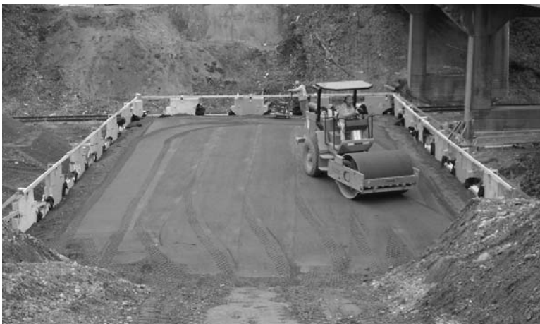
Figure 2-10. Compaction of the reinforced wall fill.
