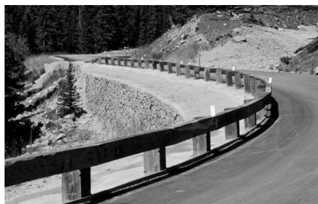
Figure 2-23. Guanella Pass architectural concrete faced wall.
