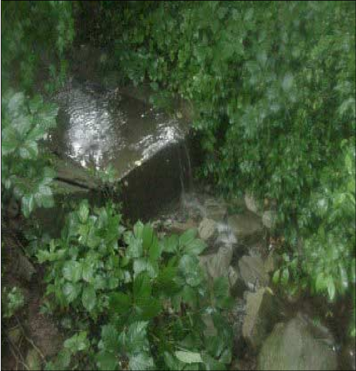
Figure 16. Sampling point N255 at end of concrete channel.
