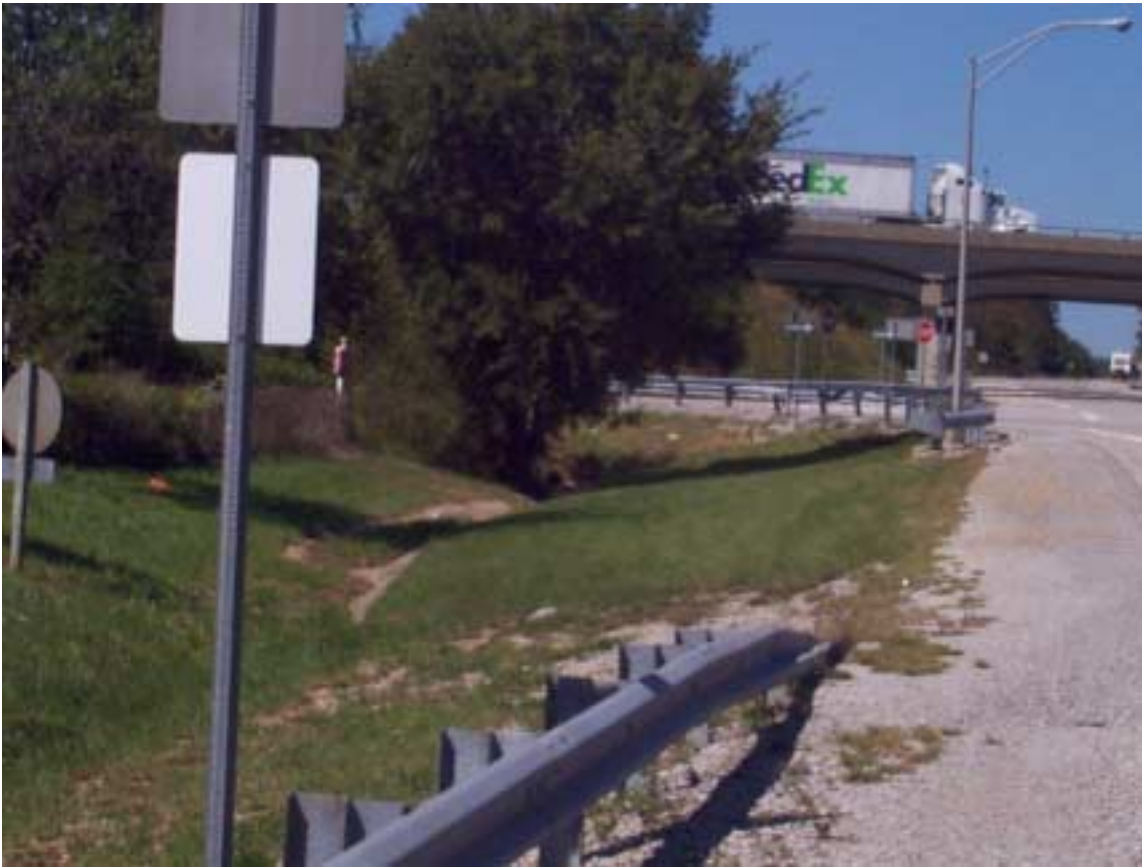
Figure 17. Concrete lined channel on south side of KY 255.
