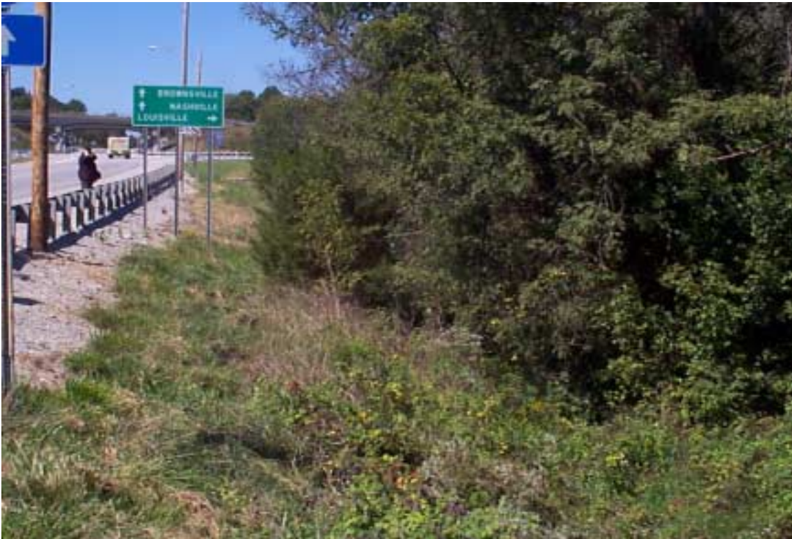
Figure 15. Lined channel covered with brush north of KY 255.
