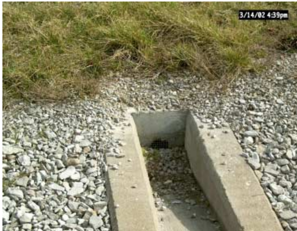
Figure 8. Drainage under I-65 to prevent highway flooding.
