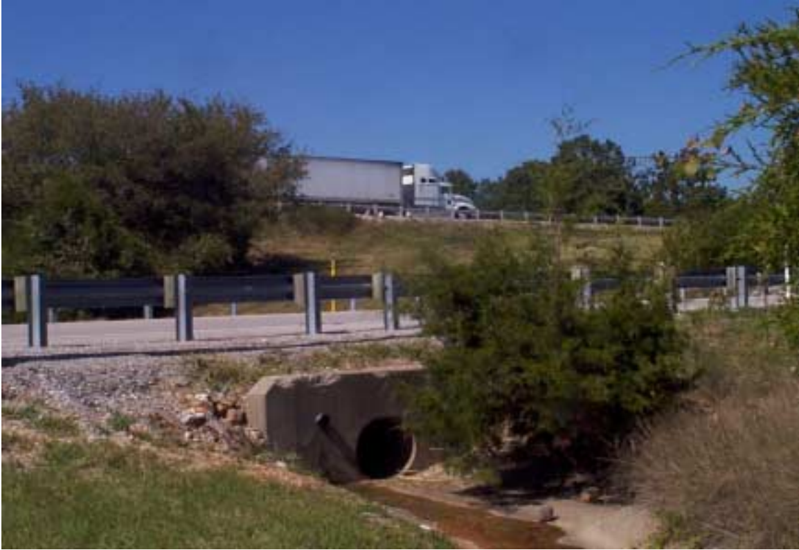
Figure 10. Drainage under ramp to I-65 north.
