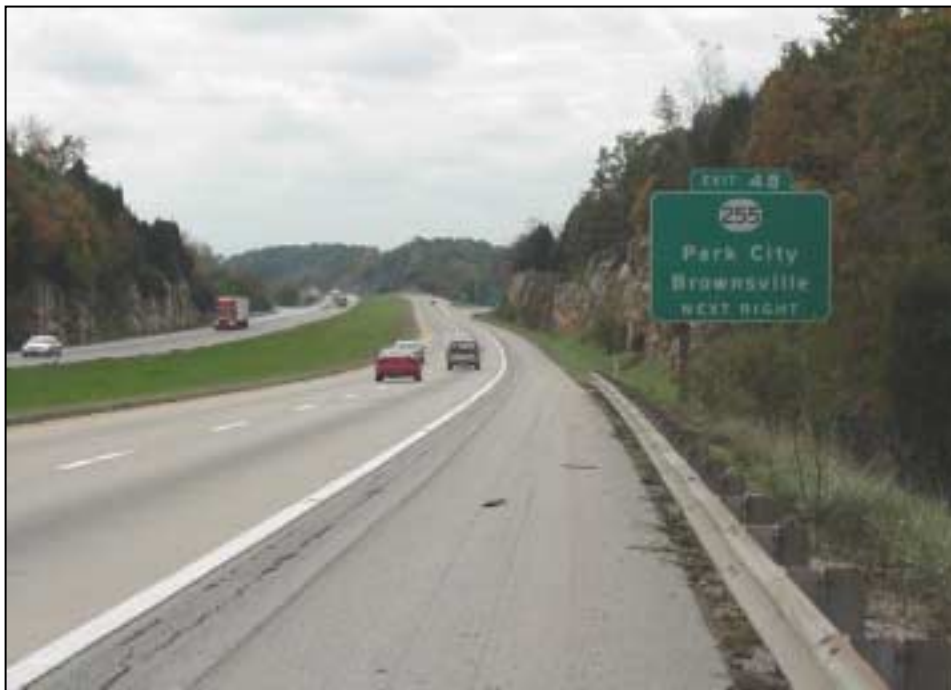
Figure 5. I-65 looking south at exit ramp for Park City.
