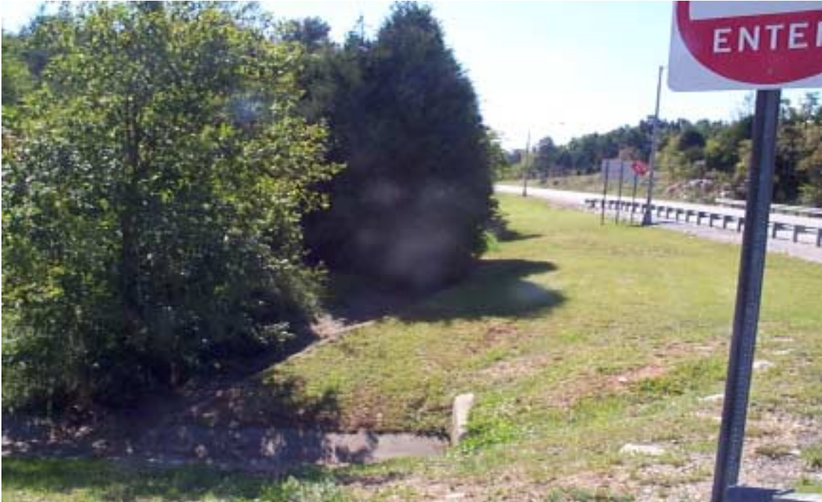
Figure 19. Concrete lined channels on east of I-65.
