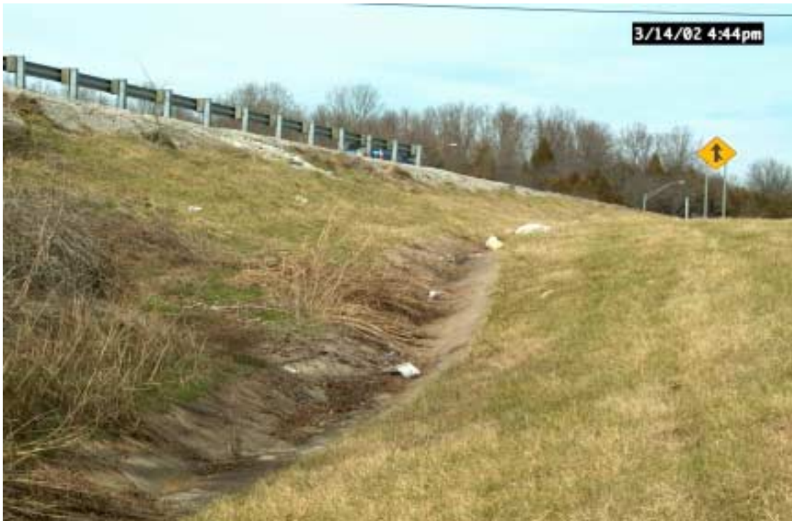
Figure 21. Concrete lined channel on east of I-65 N.
