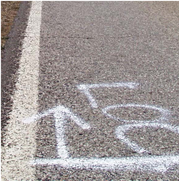
Figure 3.16 Chip sealed pavement at Mountain Home site
