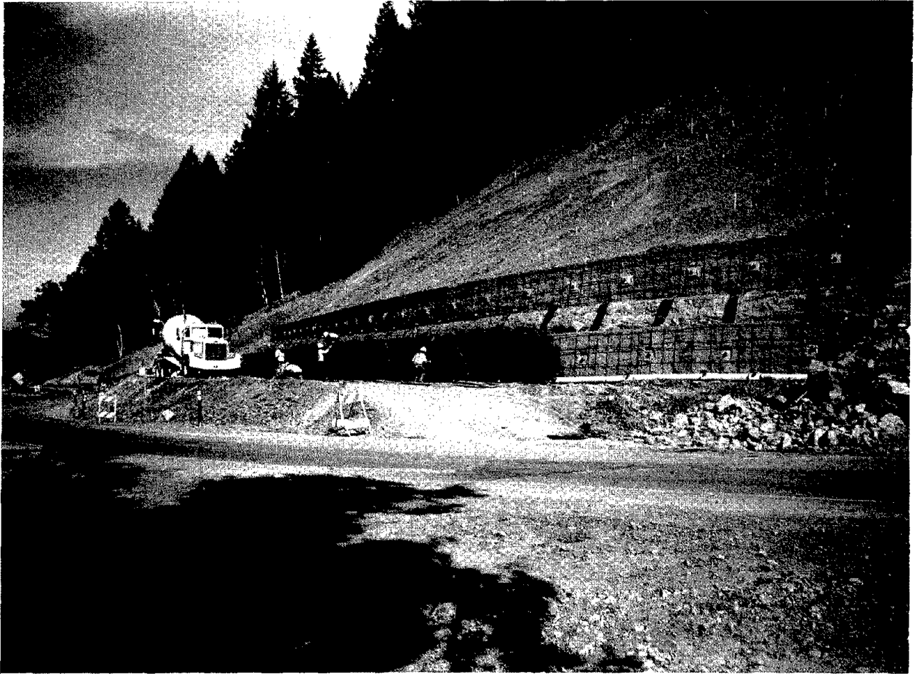
FIGURE 11 Landslide Stabilization Using Anchored Horizontal Wales for State Highway 36 in Trinity National Forest, California
