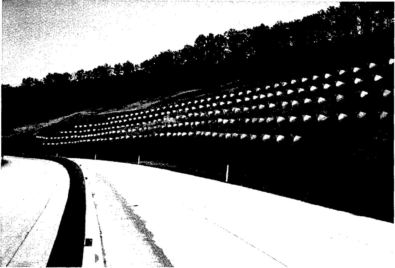
FIGURE 18 Landslide Stabilization Along U.S. 220 Near Altoona, Pennsylvania
