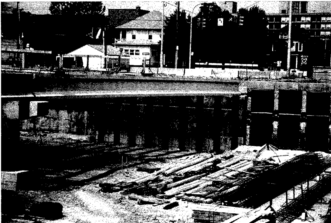
FIGURE 12 Anchored Wall and Bridge Abutment Under Construction on Davidson Freeway, Detroit, Michigan
