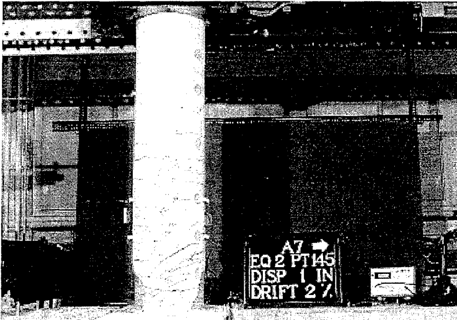
FIGURE 5-4 Damage to Specimen A7 at Half Cycle No. 145 During Earthquake #2
