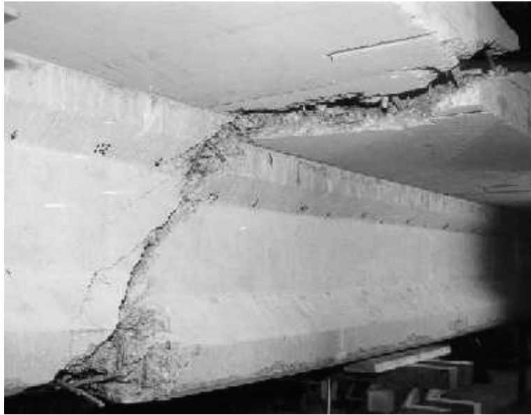
Figure 8.4 Second End Region Shear Failure of the Specimen WNEP
