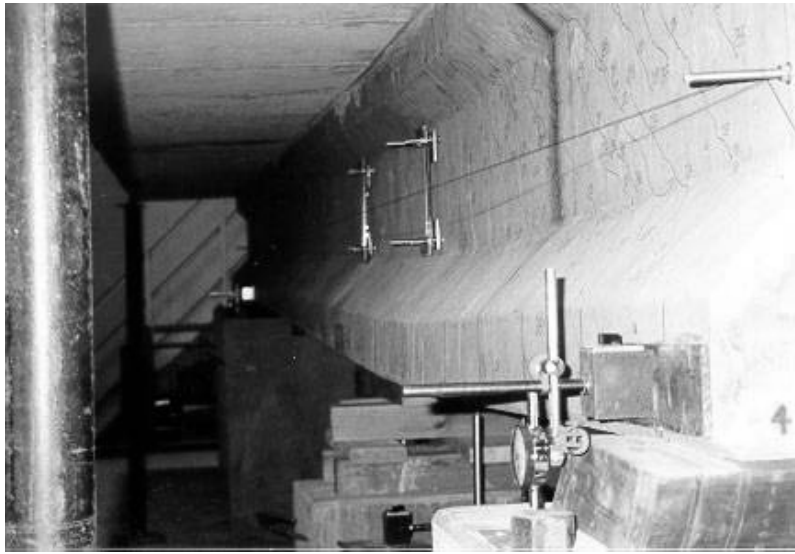
Figure 4.2 Wire Gage Deflection Device
