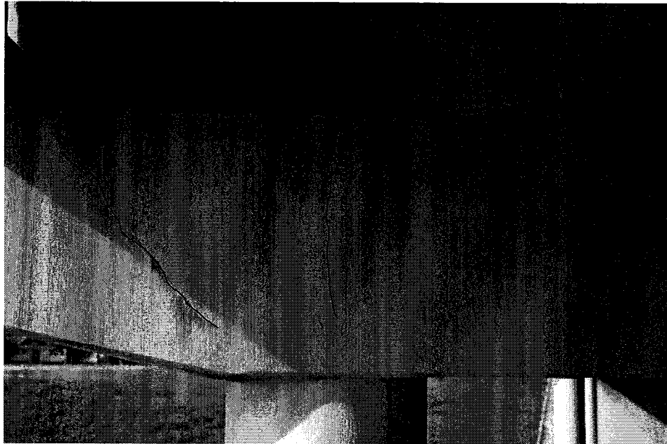
Figure 4.1. Typical Field Observed Cracking Pattern.
