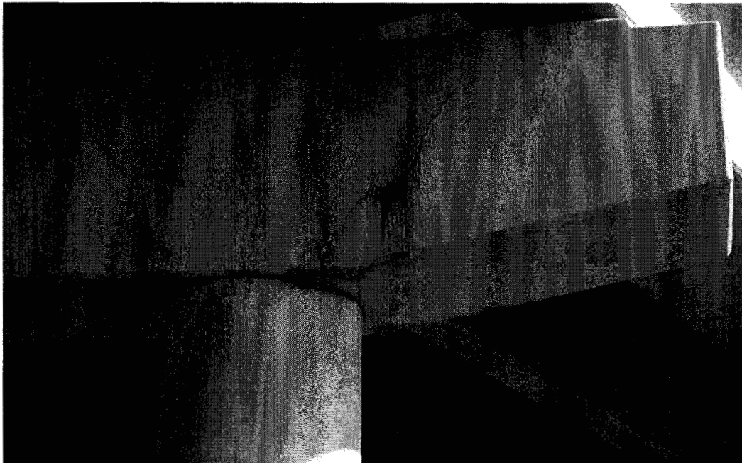
Figure 2.1. Cracking in TxDOT Bent Cap at the Cantilevered End, View #1.
