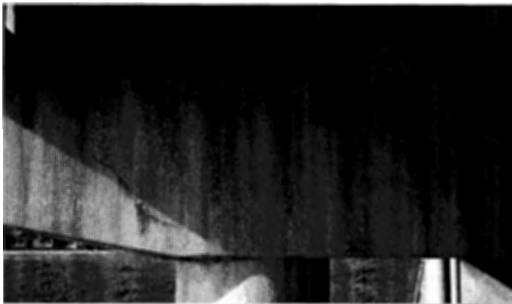
Figure 2.2. Cracking in TxDOT Bent Cap at the Cantilevered End, View #2.
